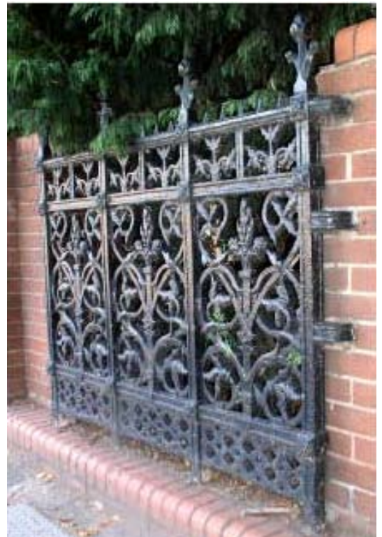
Sections of the original cast iron railings have been incorporated into the modern boundary wall at 119 Loughborough Road.
