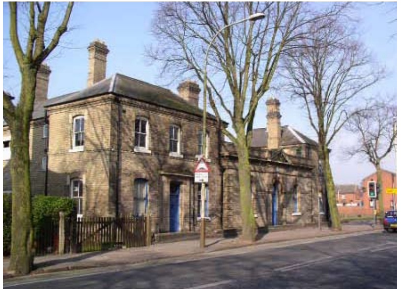
The former Police Station, 176-180 Loughborough Road, is one of the few buildings constructed from cream bricks. The frontage consists of a single storey central section and two corner blocks with pavilion style roofs.
