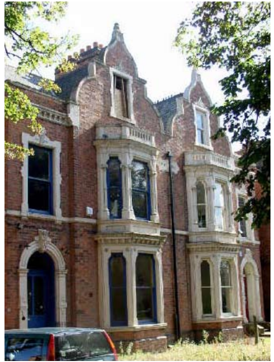
These two properties at 115 and 117 Loughborough Road have impressive Dutch-style gables and date from the 1870s. The original windows and doors are encased in stone in a style known as 'Gothic Revival'.
