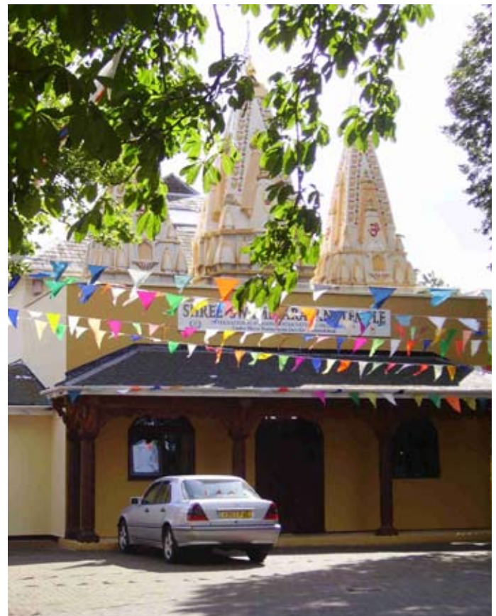
The Shree Swaminarayan Temple at 139 Loughborough Road. Since the original appraisal of 2003 the attractive brightly painted wooden porch has unfortunately been re-painted in a dark brown colour.
