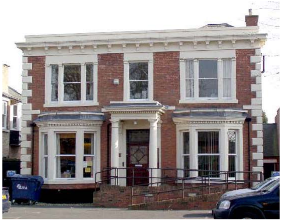
Many of the grander properties such as 131 Loughborough Road have elaborate windows and door surrounds constructed from stone.
