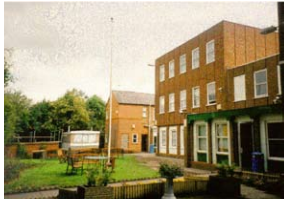
The flat-roofed 1970s extension to 119 Loughborough Road is of poor architectural quality and detrimental to this part of the Conservation Area.
