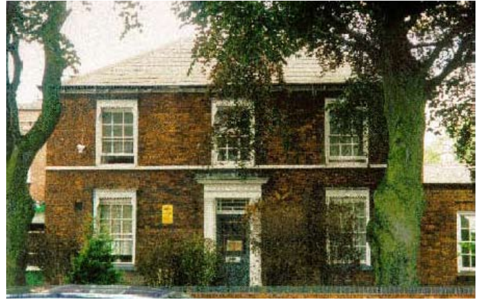
Penn House, 119 Loughborough Road is the earliest building within the Conservation Area.
