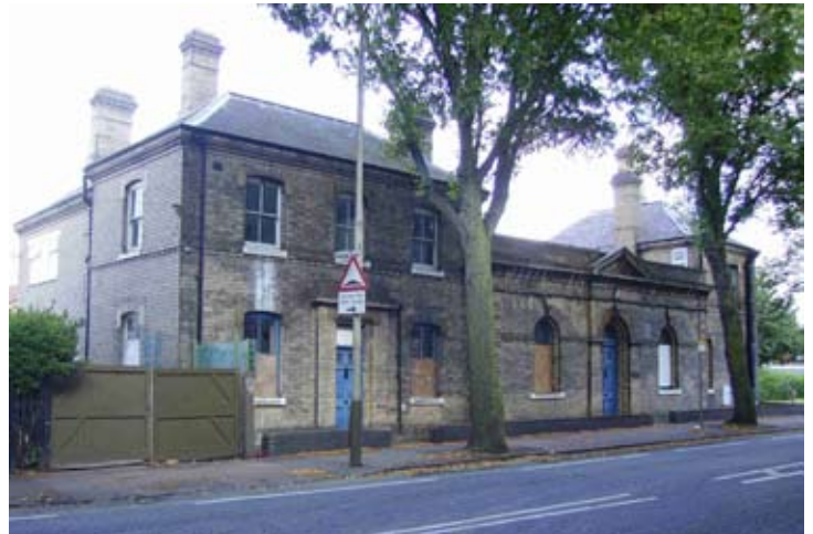
The former Belgrave Road Police Station near to the corner of Holden Street.
