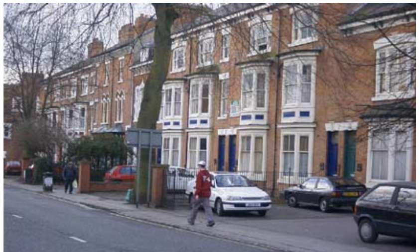
The loss of front boundary walls and gardens to provide space for car parking along Evington Road has caused a major loss of character to this part of the conservation area.
