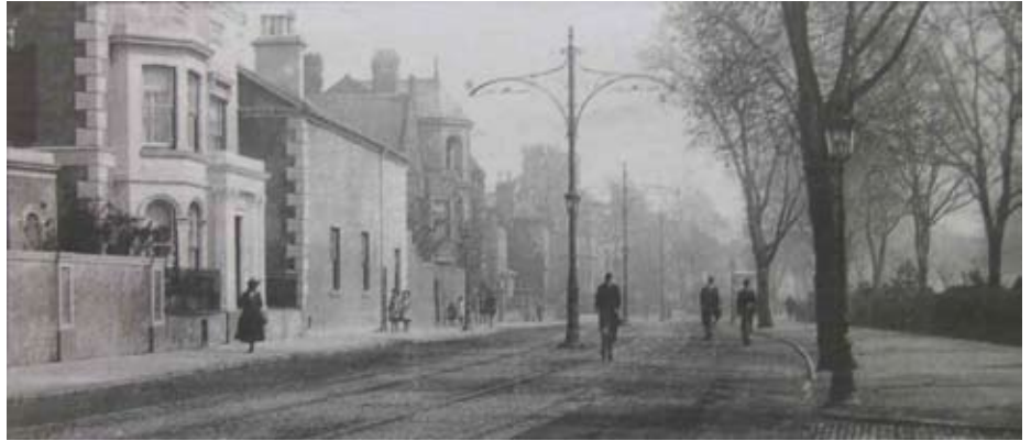
Above: Two historic views of London Road c 1904 showing the ornate cast iron supporting columns and structure of the newly installed tramway system. The building to the far left of the lower picture was known as Granby House (158 London Road), it was demolished during the 1970s
