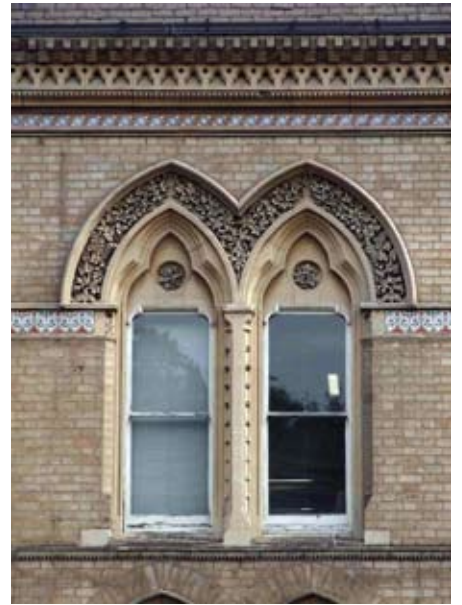
Rich ornamentation on London Road. The deeply carved window arches are as fine as those on the best medieval churches.
