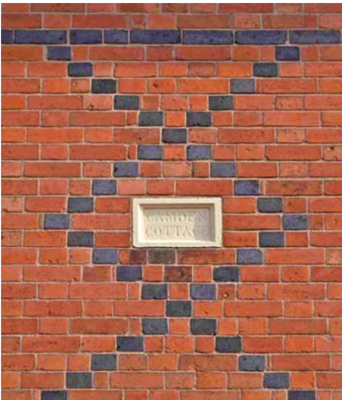
Number 4 St. James Terrace: blue brick diaper work, set around a small stone plaque
