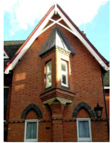
Gable detail to the Old Vicarage, at 11 St. James Road.
