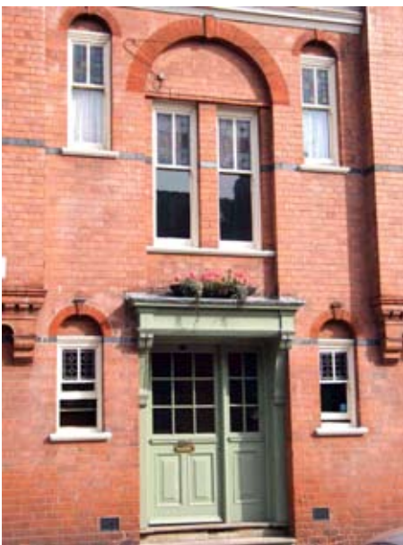
Detail of entrance to 2 Chaucer Street.
