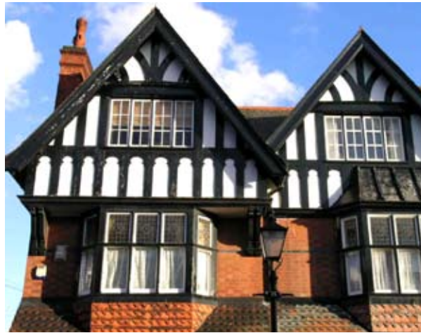
Gables to 1 Tennyson Road and 31 St James Road.
