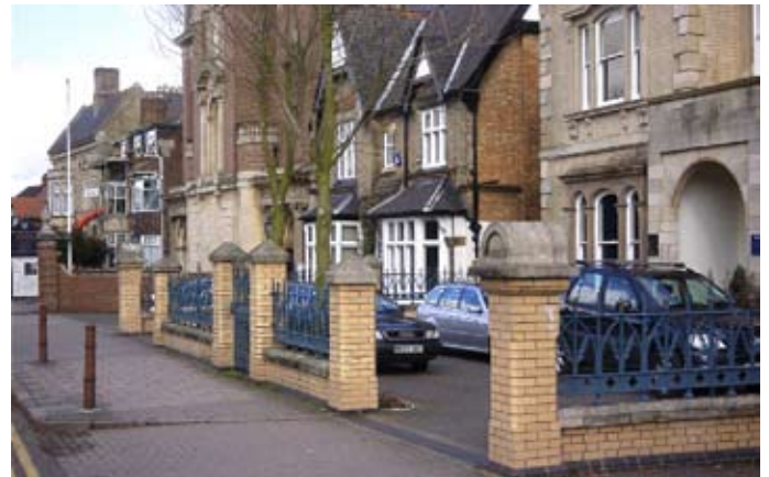
The use of "angel-wing" style railings at 218 London Road.
