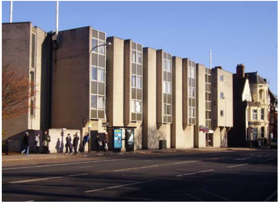
The four-storey block of apartments at 158 London Road suffers from the loss of the rear boundary wall to Evington Footpath to allow access for car parking. The lack of any boundary treatment to the London Road frontage is also unfortunate and has resulted in a sterile feel to the immediate surroundings this block.
