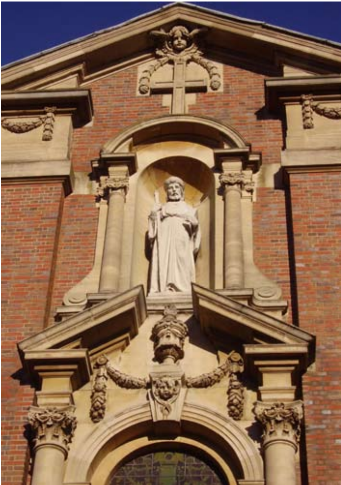
Detail of the broken pediment to the west front of St. James the Greater. The figure is of St. James.
