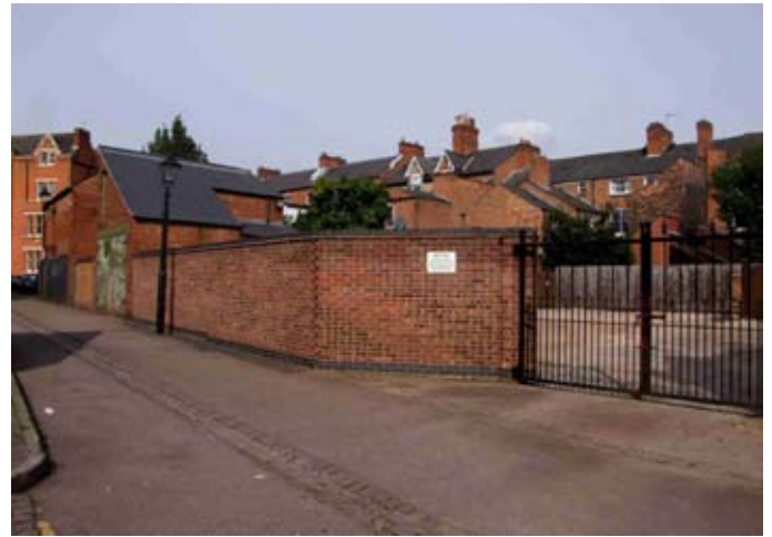
The Footpath at the northern end showing the parking area opposite the flats at 158 London Road.
