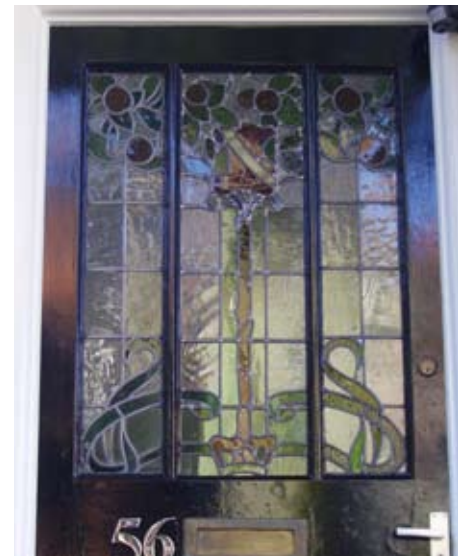
Many of the fine houses on St James Road survive with all their features, including highly decorative stained glass door panels
