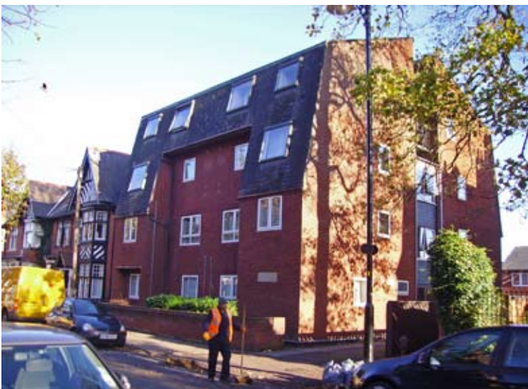
The overall design and excessive scale of 13-17 St James Road does nothing to complement the rest of the residential properties nearby.
