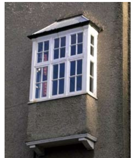
First floor oriel window to the St James Road elevation of 202 London Road.
