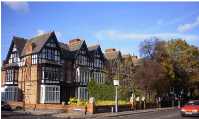
Trees along Narborough Road, protected by a Tree Preservation Order, in front of the imposing terrace of 169-195
