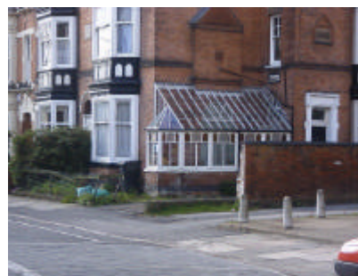
Loss of front garden walls and storage of wheelie bins in front gardens have eroded the character of the area.
