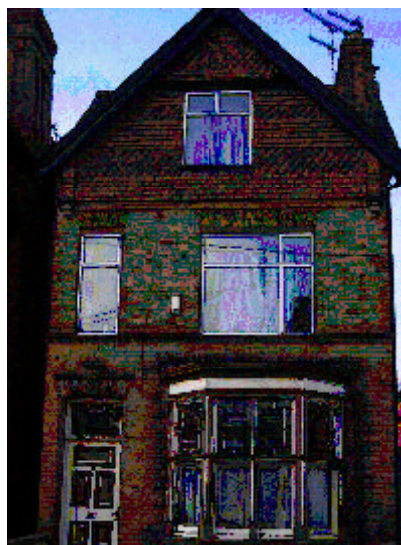
Replacement windows such as these in the upper floors began to eat away at the special character of the area and created the need for the Article 4 Direction
