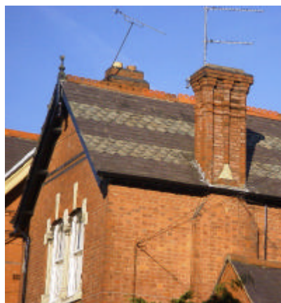
Distinctive Welsh slate roof with bands of fish scale and red clay ridge tiles with terracotta finials are relatively common features within the area and used throughout the 169-195 Narborough Road terrace.
