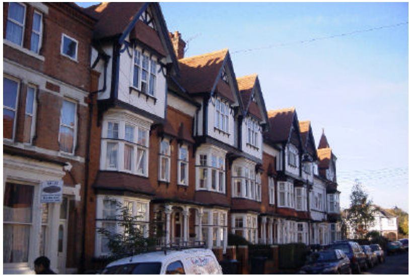
Large terraces on Westleigh Road
