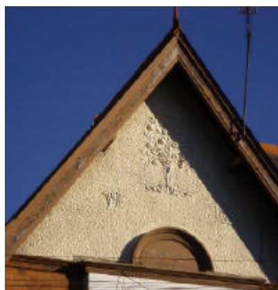
Pargetting on the gable of the nursing home, 19 Ashleigh Road
