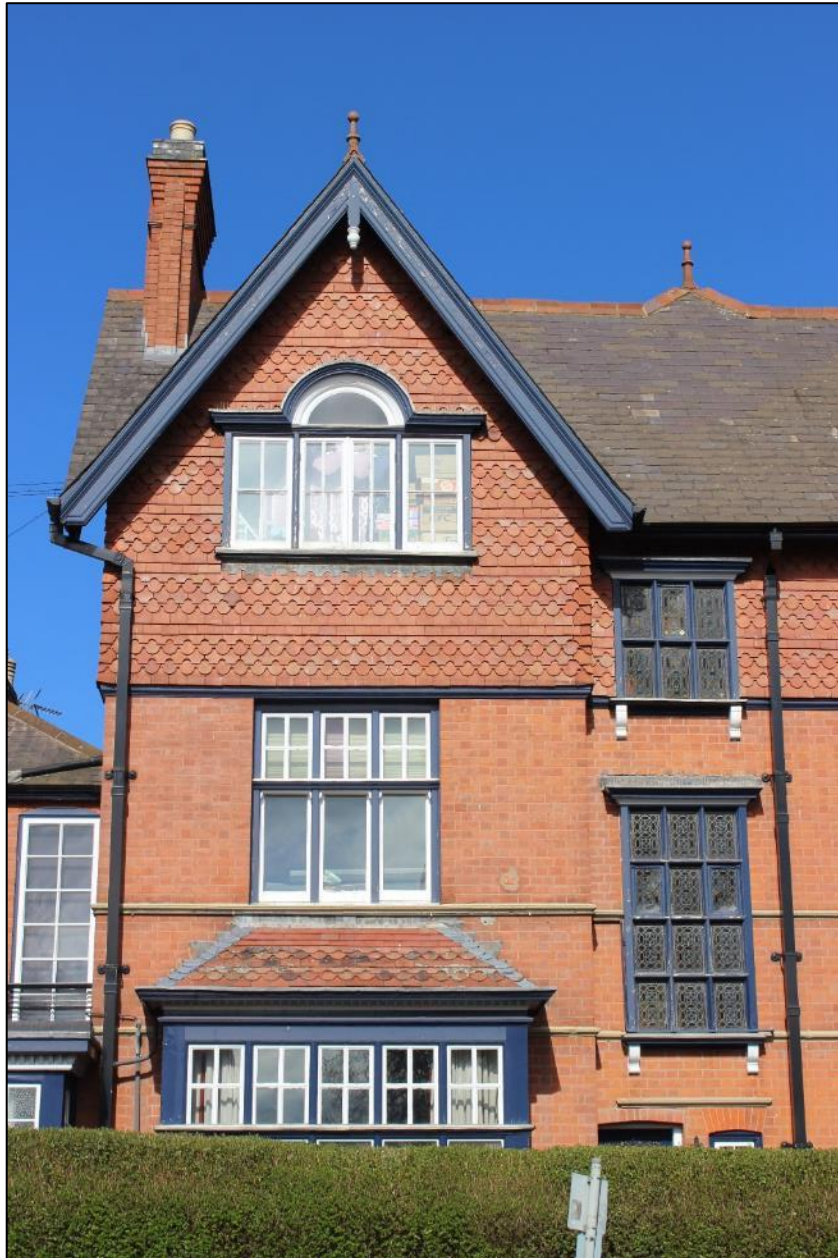
Figure 49: Woodgate House at 37 Fosse Road Central is constructed of the common Leicester red brickwork, with hanging tiles commonplace throughout the Conservation Area.
