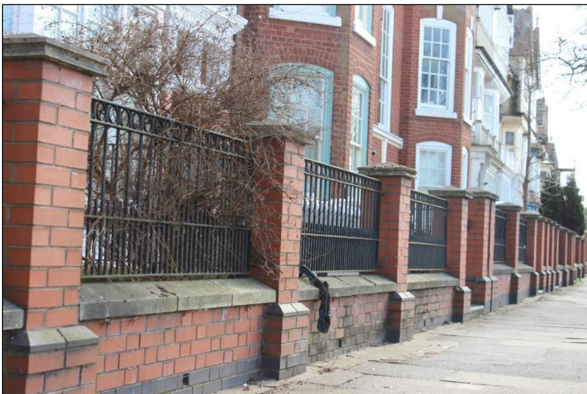
Figure 57: The reconstructed modern front boundary walls with railings along Fosse Road South, with some of the original capping stones retained.
