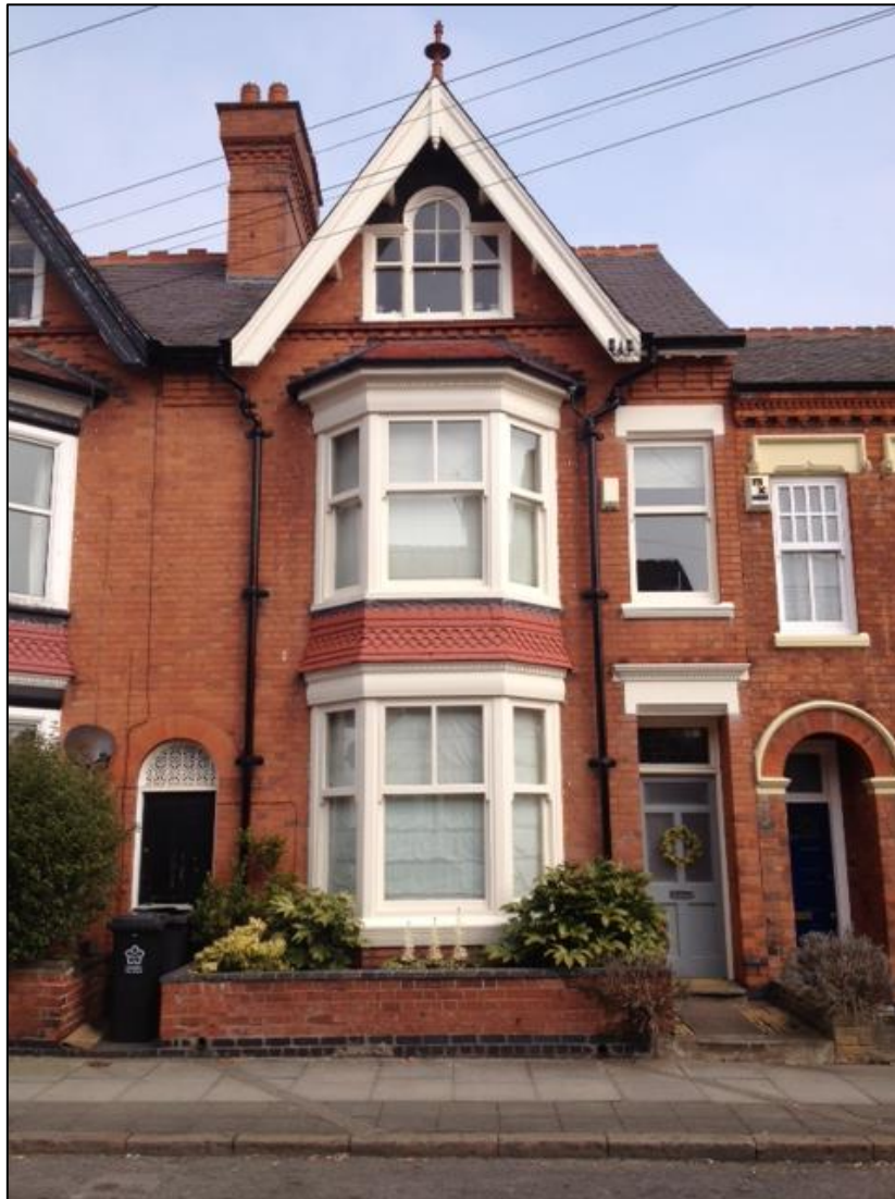
Figure 23: The house at 51 Stretton Road, with a Venetian window to gable and hanging tiles to full height canted bay.
