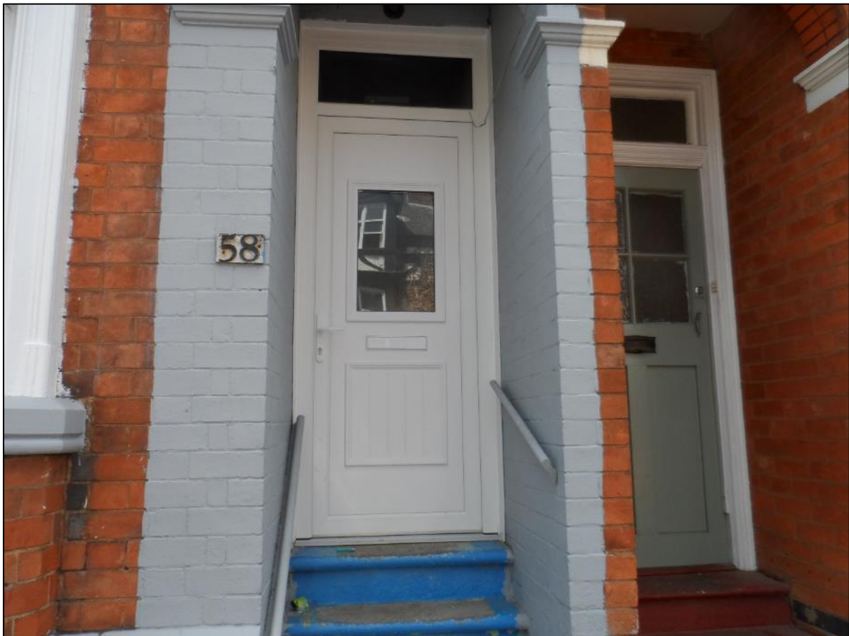
Figure 64: The plastic (uPVC) door recently installed at 58 Stretton Road failed to preserve the character of the historic property and replicate the quality and design of the original door.
