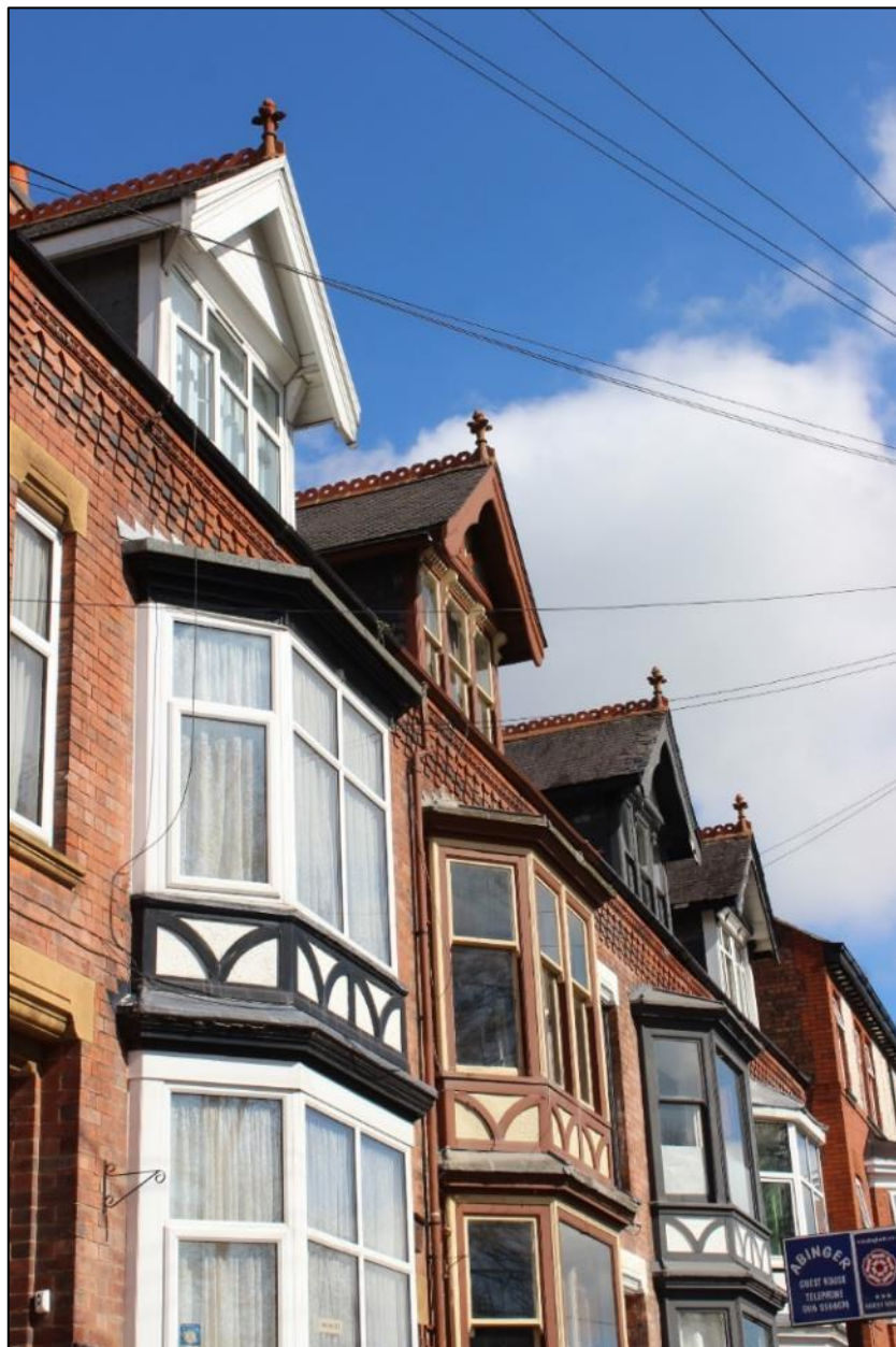
Figure 28: Dwellinghouses at 171-175 Hinckley Road, with half timbering to canted bays.
