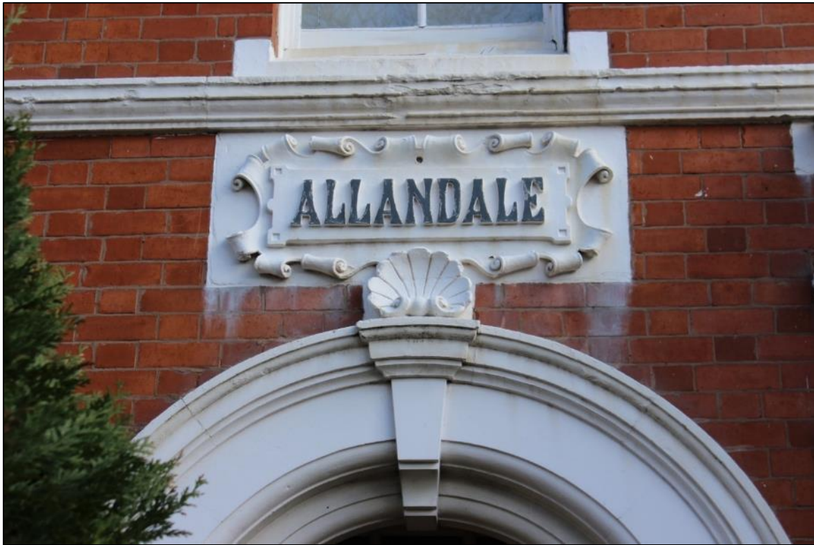
Figure 33: The carved name plaque at 10 Fosse Road South, above a stylized keystoned archway topped with a stylized shell.
