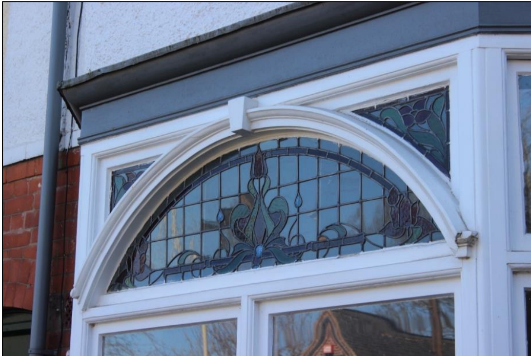
Figure 40: The original moulded joinery and stained glazing at 96 Westcotes Drive.
