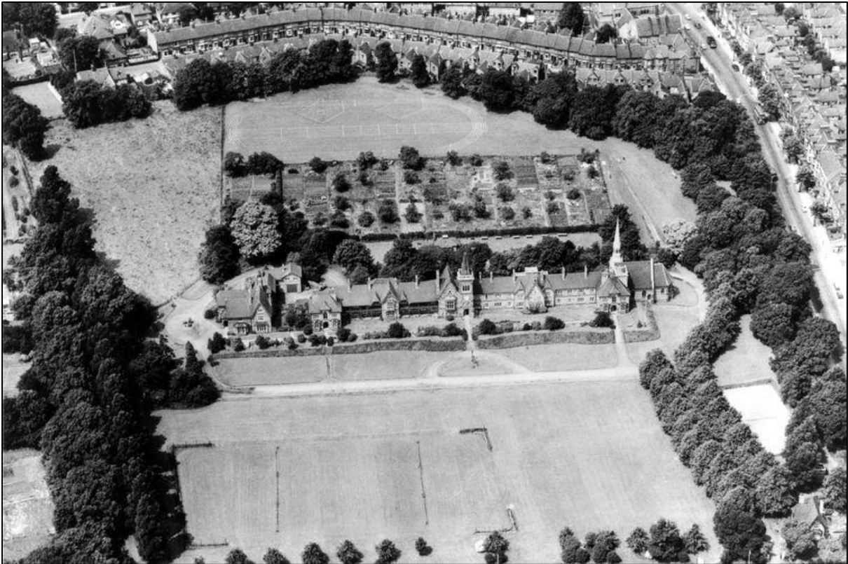
Figure 4: A view of the old Wyggeston's Hospital built in 1868, c.1960.
