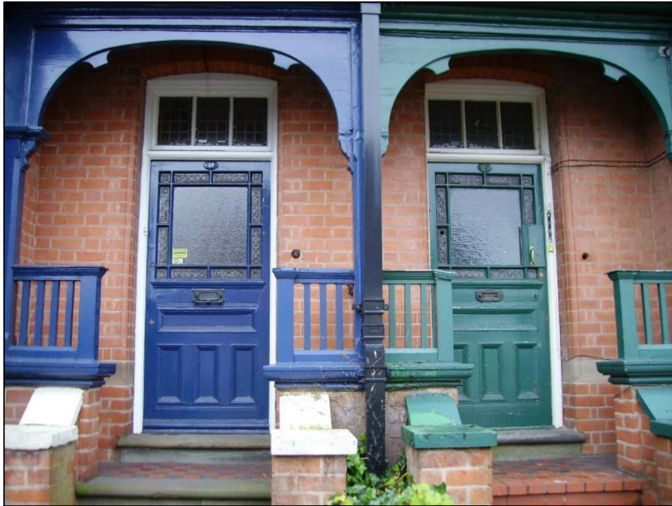
Figure 19: The original doors and porches at 33-35 Fosse Road Central.
