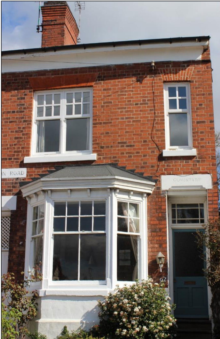
Figure 30: The frontage of the dwellinghouse at 82 Dulverton Road, with some original joinery still intact.
