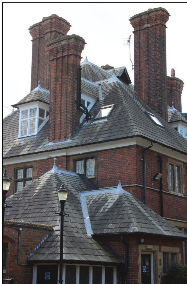
Figure 53: The Cumberland slate hipped roofs at the Grade II Listed Sykefield.
