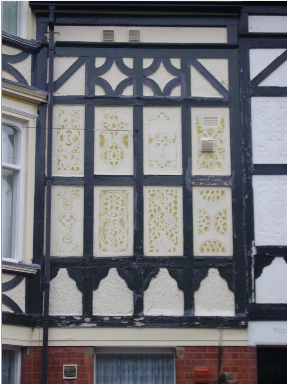
Figure 24: Sham timber framing and pargetting at number 81 Stretton Road.
