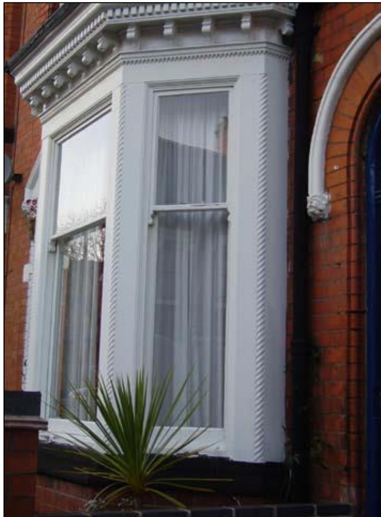
Figure 22: Detail of 1 Stretton Road, showing 'barley-sugar' twists to the corner mullions of the splayed bay windows.
