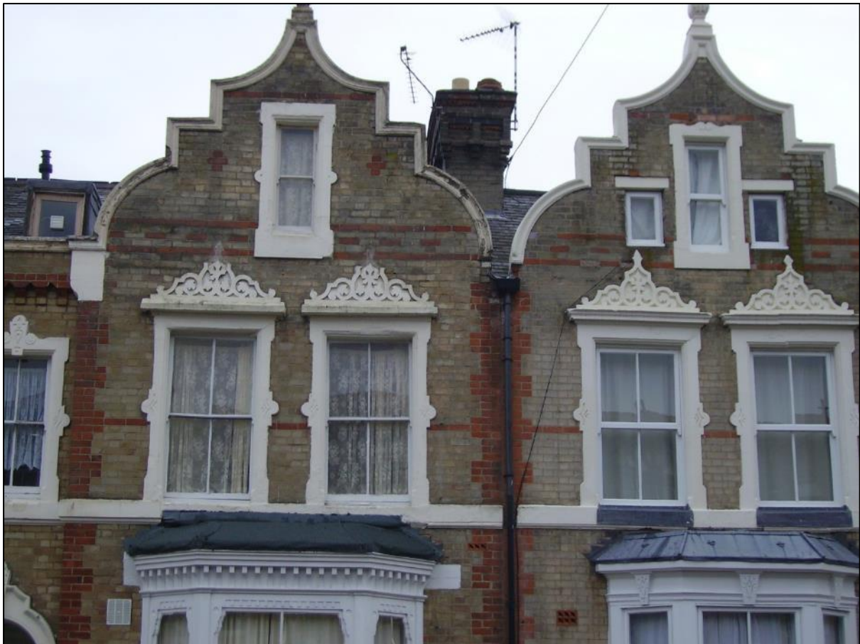
Figure 50: The buff brick properties at 42-48 Fosse Road Central, with stylized Dutch gables and stucco detailing.
