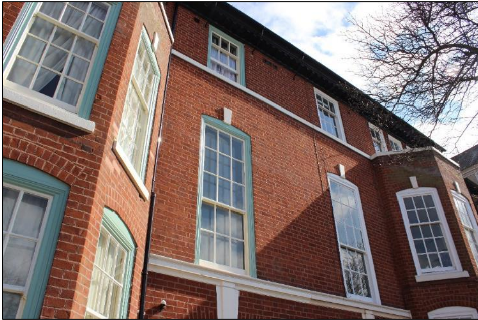
Figure 35: The three-storey neo-Georgian building at 22-24 Fosse Road South, with original tall sash windows under keystone arches.
