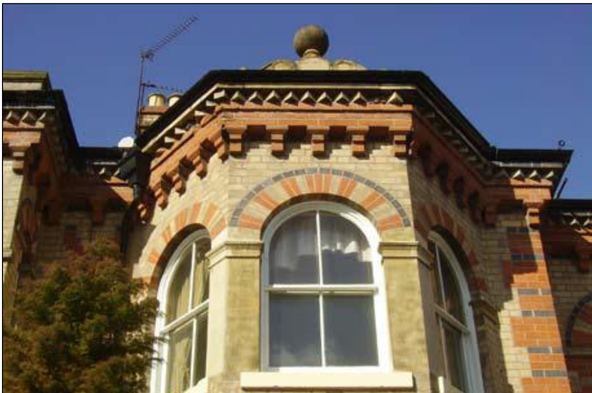
Figure 17: A detail of the first-floor bay to what was originally 'Dane Hill Villa' showing some of the red and white polychrome brickwork, characteristic of a number of buildings in the Conservation Area.
