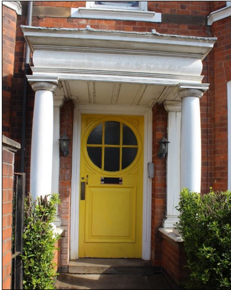
Figure 59: The timber and stone portico supported on Tuscan columns and the original solid timber door with circular glazing.
