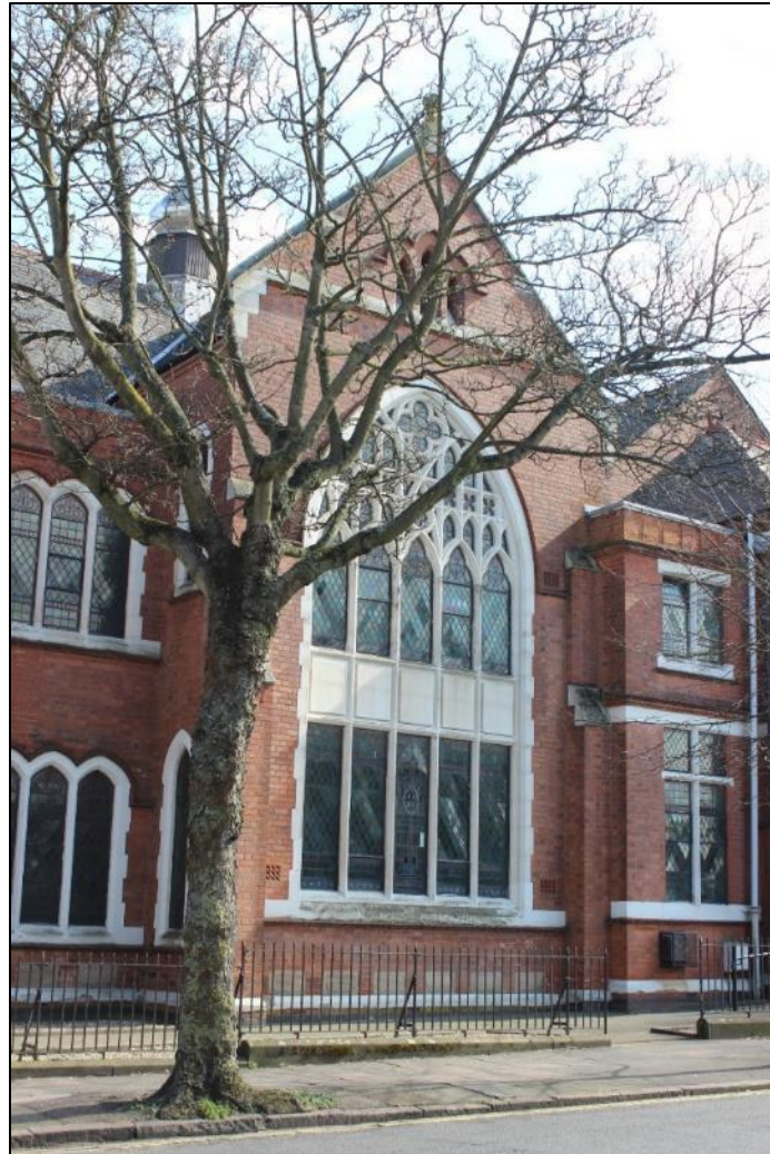
Figure 31: Gothic Revival windows to the side elevations of the Ukrainian Catholic Church, constructed in 1898 as the Primitive Methodist Chapel.
