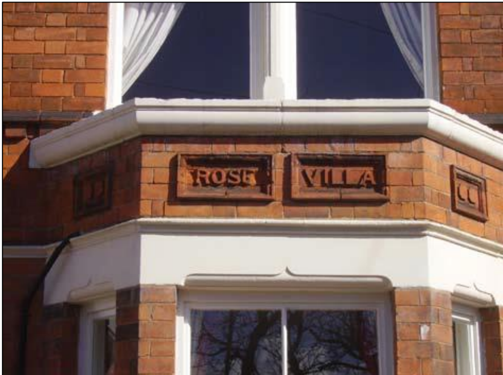
Figure 21: Decorative moulded brick detailing to the angled bay of 33 Stretton Road (Rose Villa).
