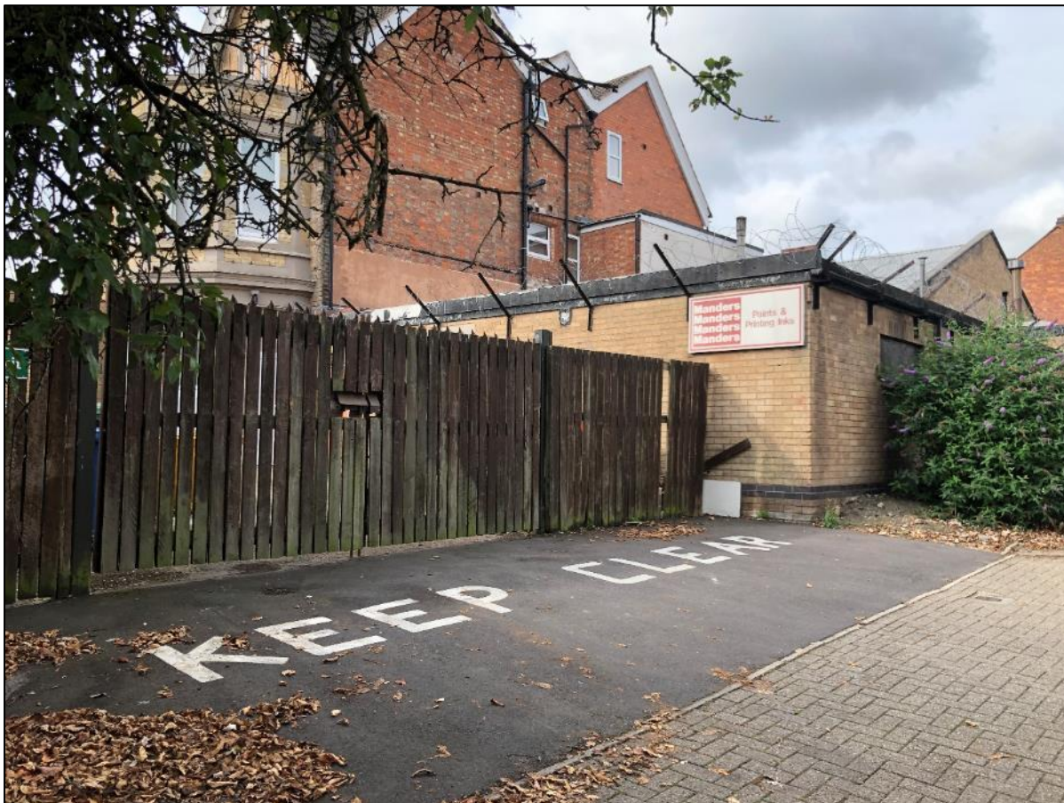
Figure 66: The rear of the properties at 125-137 Hinckley Road is in poor condition, with a tarmacked driveway and poor-quality fencing.
