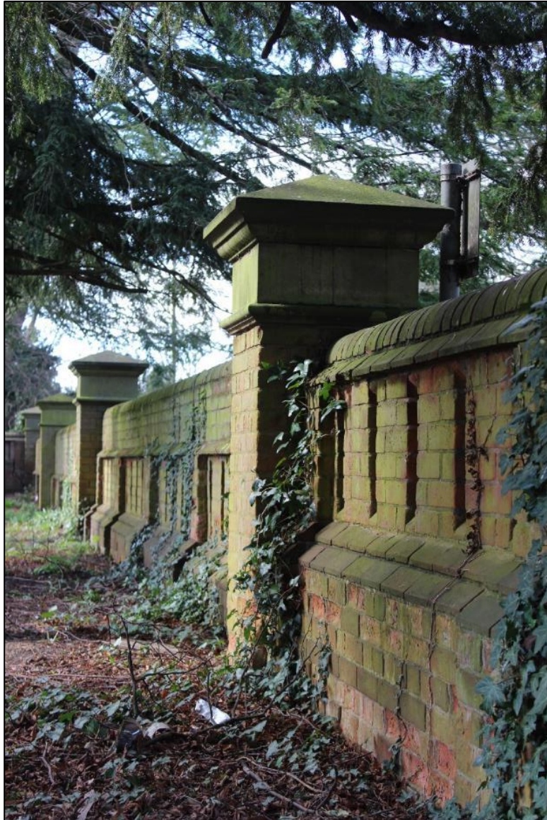
Figure 56: The Grade II Listed brick walls and gate piers to Sykefield.
