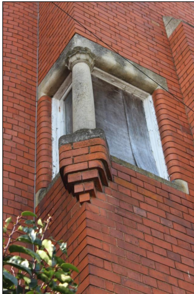
Figure 41: The unique brick and stone decoration at the corner of the Art Nouveau Bradgate House.
