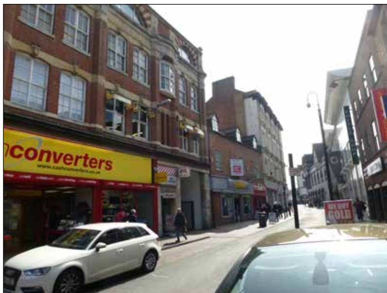
The dramatic juxtaposition between the 18th century 9-11 Church Gate and the adjacent later buildings is evident and creates a strong sense of place.
