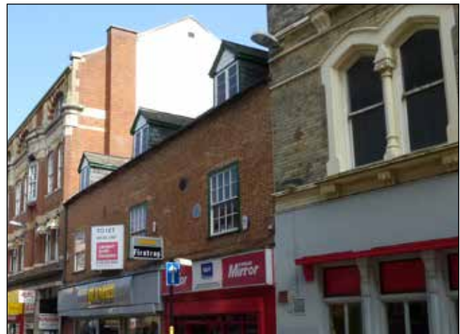
Good quality bricks laid in decorative patterns helps form a strong positive character for the area and contribute towards its local distinctiveness.
