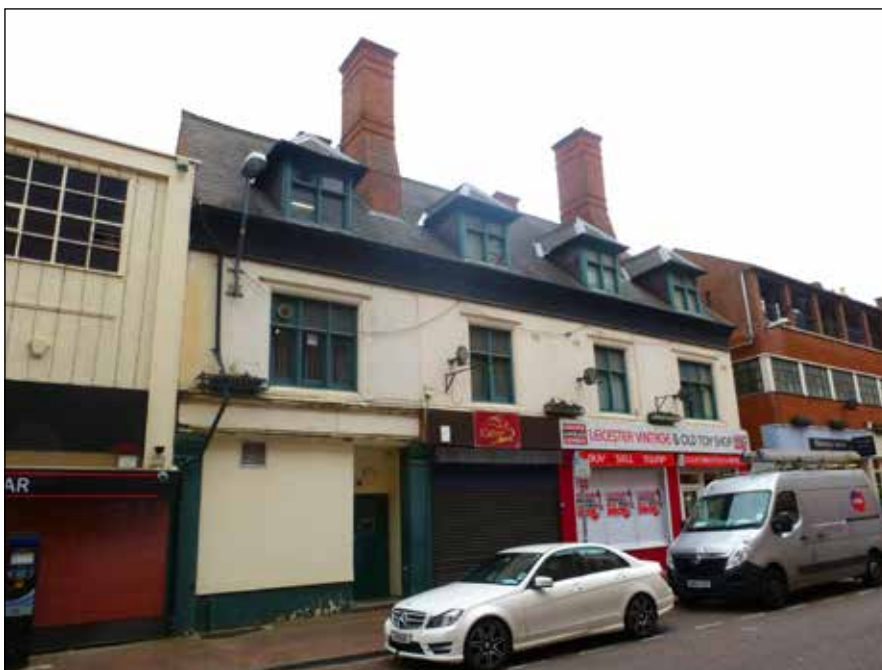
9-15 East Bond Street retains much original character.
