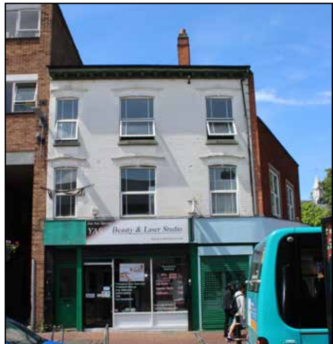
50 Church Gate is the last building in the row
