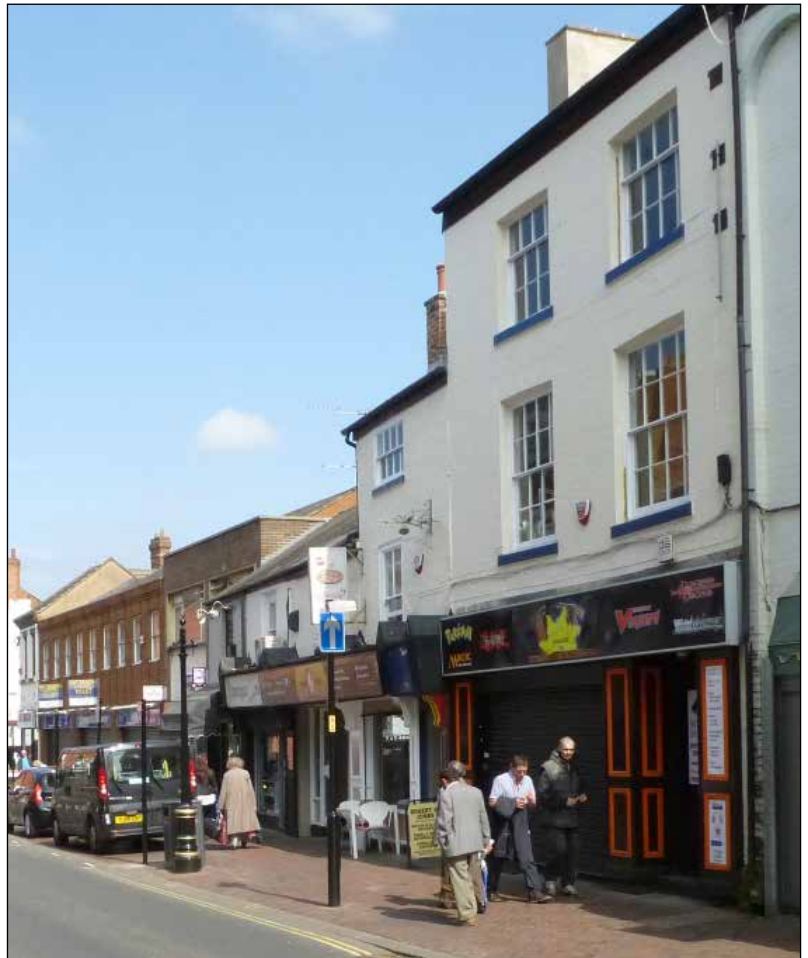
The restoration of traditional windows to the upper floors of 39-45 Church Gate has helped restore lost character and contributes greatly to the overall character of the area.
