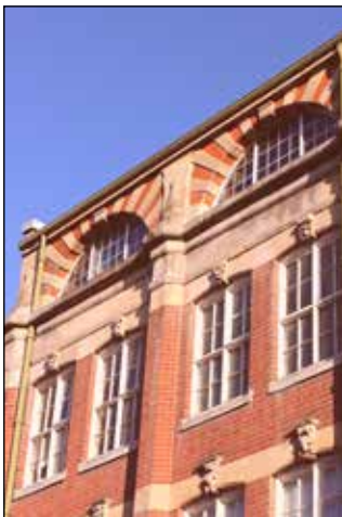
Brick and stonework on 13-21 Church Gate.
