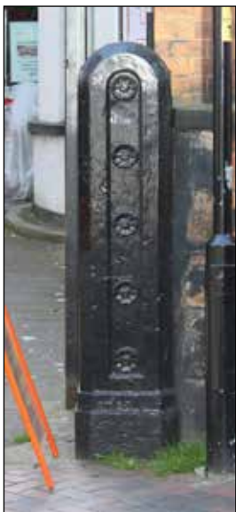
Cast Iron gate pier at 66 Church Gate.
