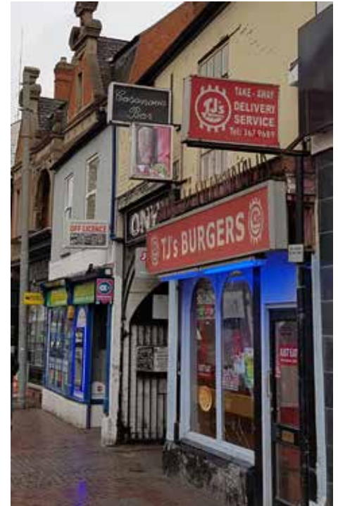
Inappropriate adverts at 67 Church Gate clutter the building.
