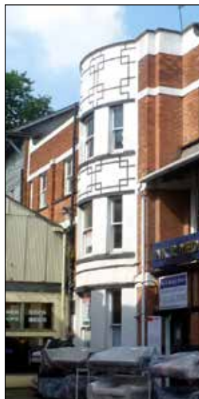
Unusual use of stucco at 66 Church Gate
