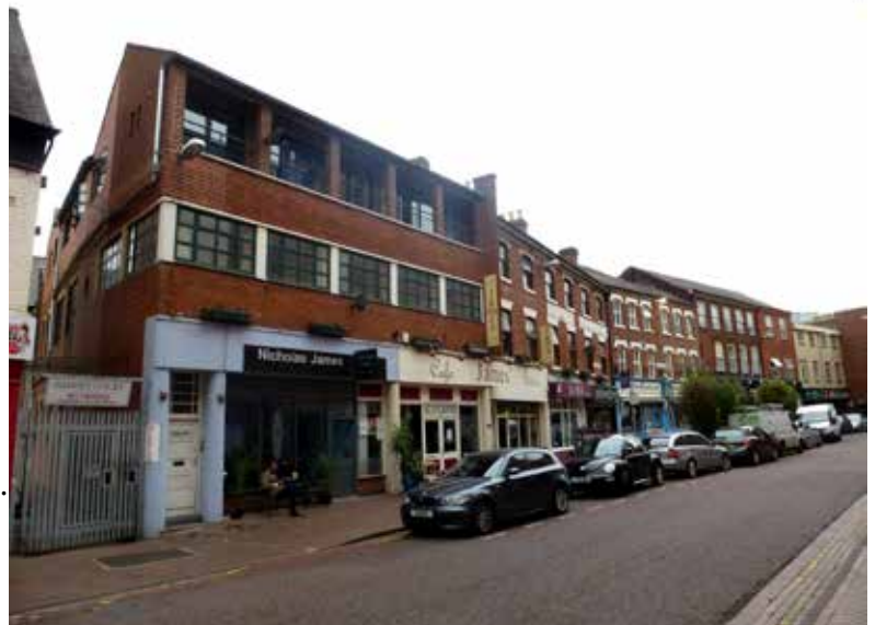
7 East Bond Street is a former vehicle garage which has been extended and converted to shops and flats.
