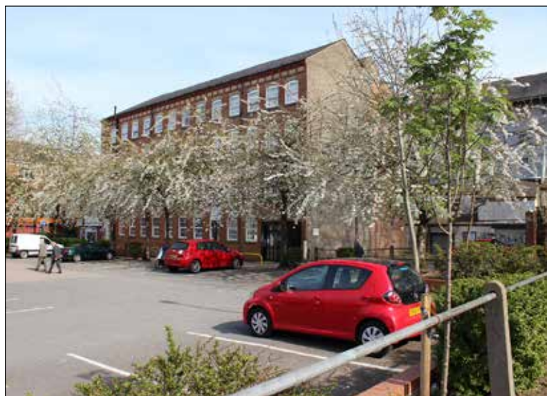
The car park serving Matalan is located on the area thought to formerly be used for Archery Butts. The site has a mixed development history, but is not harmed by being open and contains a large number of trees which make a positive contribution to the area.
