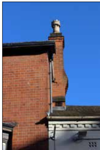
Unusual chimney detail at 27 Church Gate.
