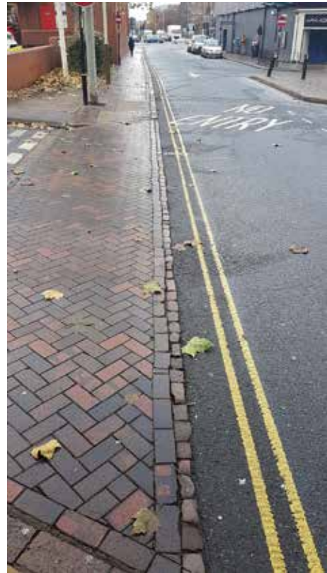
Narrow yellow lines, Church Gate.
