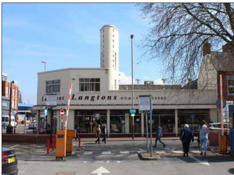
81 Church Gate is one of two former car garages in the area, the distinctive ‘fin’ forms an interesting corner feature
