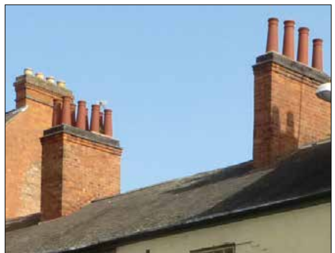
Chimneys and pots on Church Gate.
