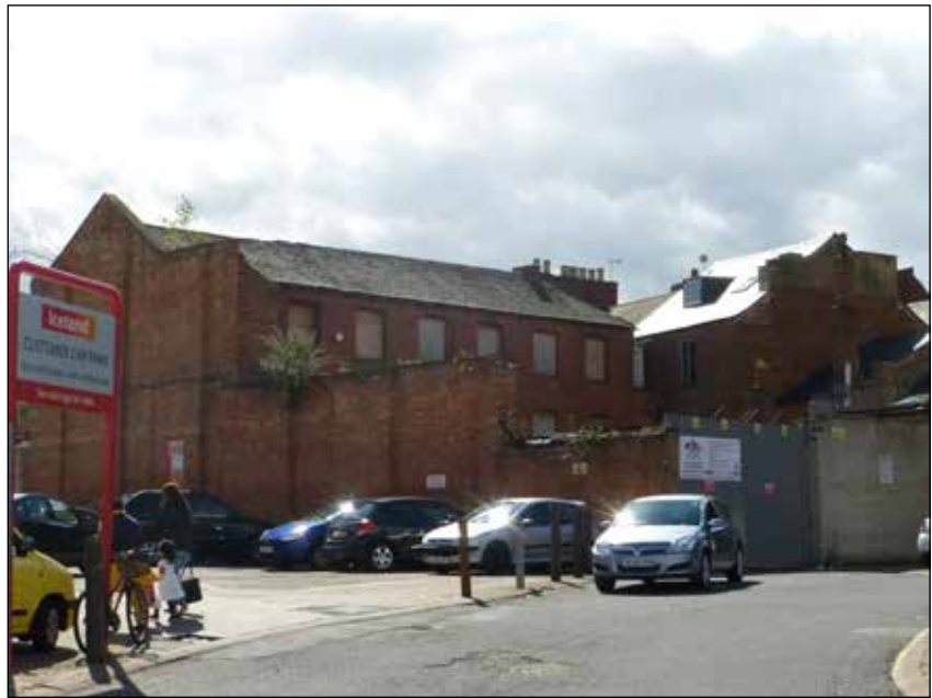
Former warehouse at rear of 39 Church Gate.
