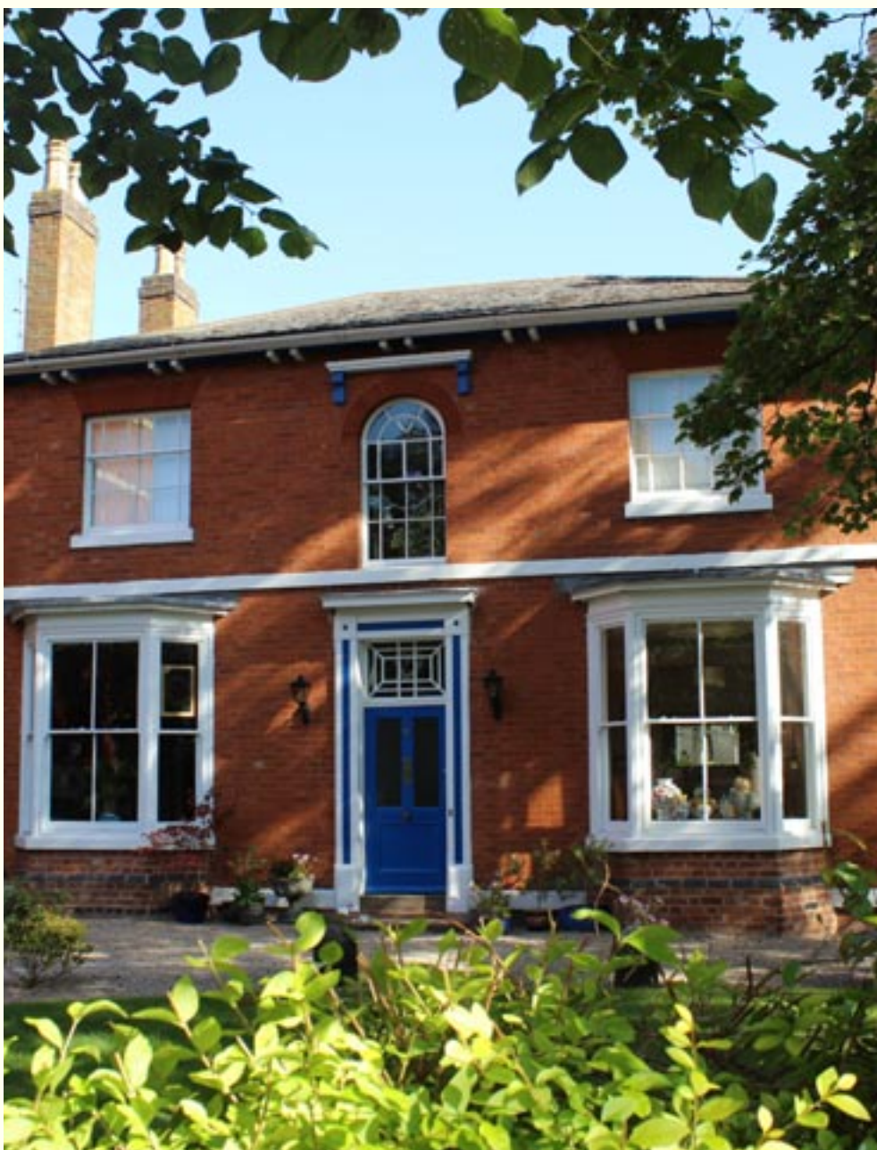
The unusual Chinese 'treslis' type fanlight above the central doorway at 72 New Walk imparts a touch of elegance to an otherwise plain facade designed in the Classical style.
