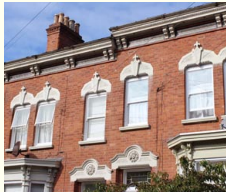
Cream clay chimney pots, decorative eaves detail, and elaborately carved stonework above the windows on West Street.
