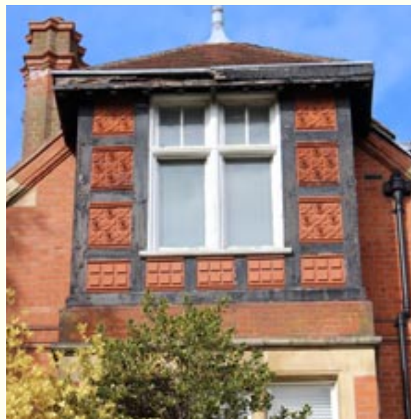
Red brick, fine terracotta moulded panels, clay roof tiles, stone and leadwork - all used to great effect on this simple hipped gable.
