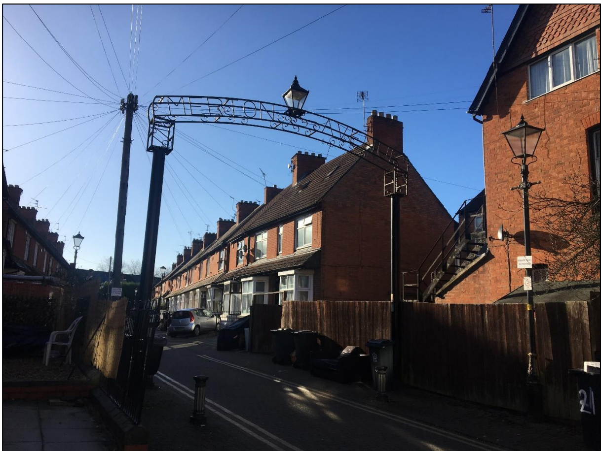
Figure 26: Formal entry onto Merton Avenue, with a decorative wrought iron overthrow on modern columns.
