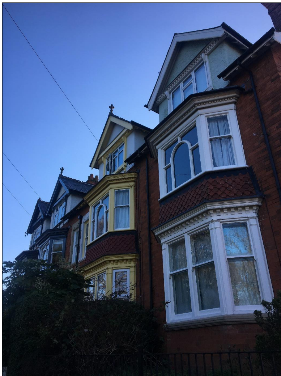
Figure 20: The dwellings at 4-6 Wentworth Road, with many of their original joinery intact.
