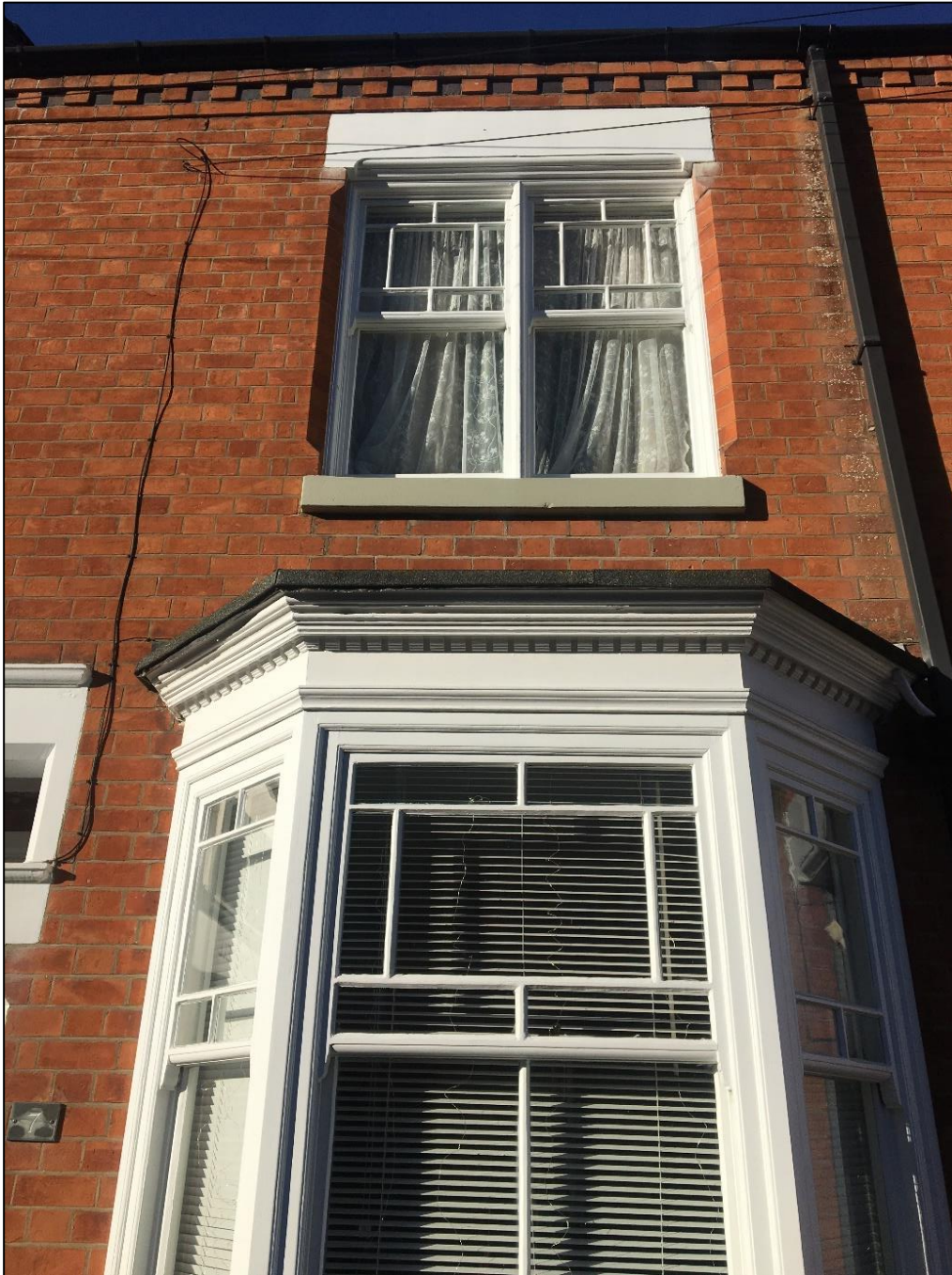
Figure 23: The original joinery to the front of the house at number 7 St Dunstan's Road.
