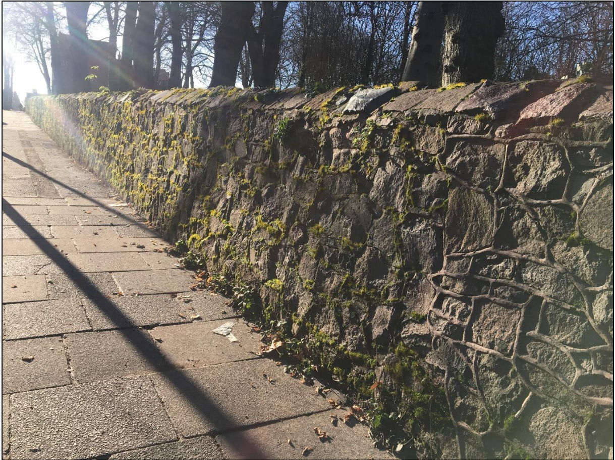
Figure 32: The Mountsorrel granite rubble walls enclose the east side of the Fosse Road Recreation Ground.
