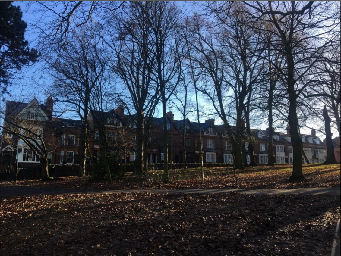
Figure 17: Terrace of historic properties at 320-344 Fosse Road North.
