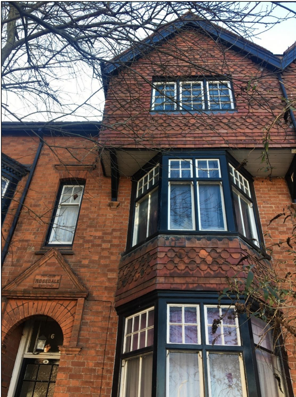
Figure 31: The hanging clay tiles and red brick elevations of the Rosedale villa make an attractive addition to the streetscene of the area.
