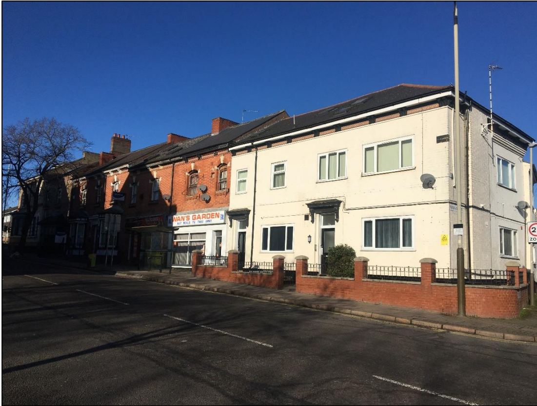
Figure 36: The painted elevations, poorly proportioned uPVC windows and satellite antennas at 21-23 Glenfield Road East have negatively impacted on the character of the area.
