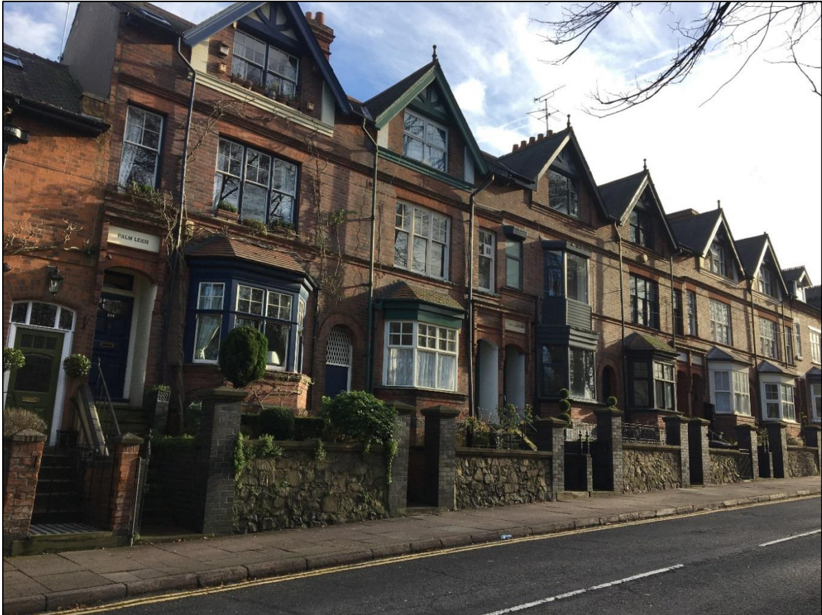
Figure 18: The canted bays and pointed gables of the dwellings at 320-332 Fosse Road North, creating rhythm in the streetscene.
