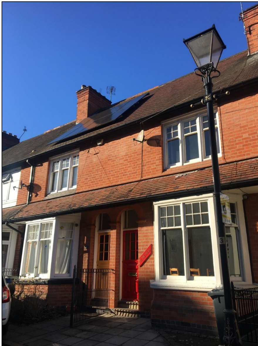
Figure 25: Merton Avenue, showing its cohesive terrace of two storey red brick artisan houses and the stylised iron lanterns.
