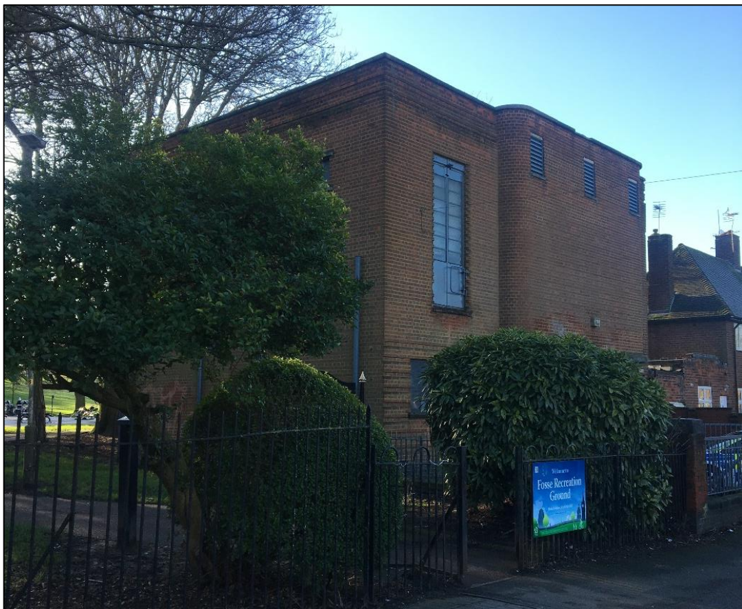
Figure 19: The 1930s electric sub-station on the north-eastern edge of the Fosse Road Recreation Ground. One of several sub-stations constructed in the inter-war period to serve the inner city and rapidly expanding suburbs, providing an electricity supply as it began to supersede gas as the main means of lighting.
