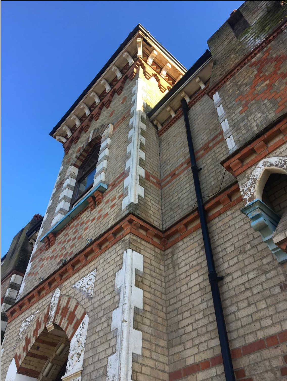
Figure 30: The buff brickwork is a somewhat unusual core building material in the area and highlights the status of the Estonian House.
