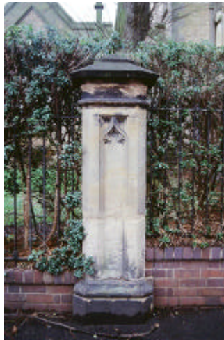
Gothic style stone pier, College Street
