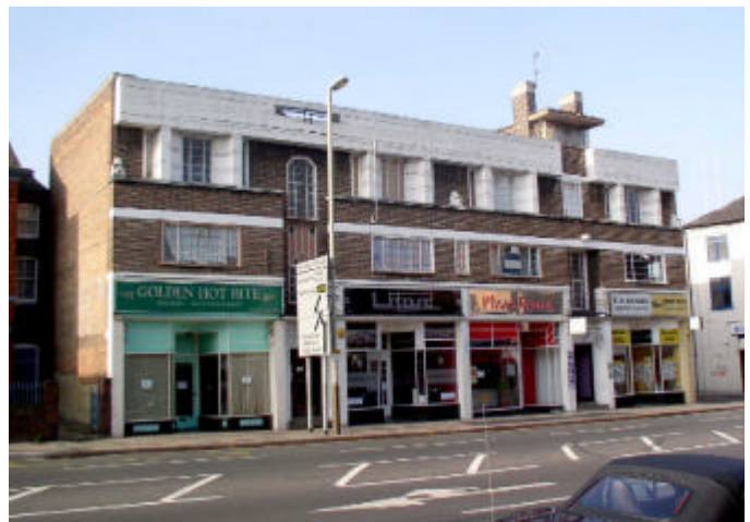
At 55 to 57 London Road there are original art-deco style shopfronts and doors.
