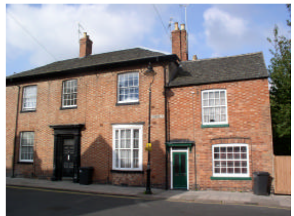
No. 20 Glebe Street and 4 Prebend Street are the earliest buildings within the Conservation Area.
