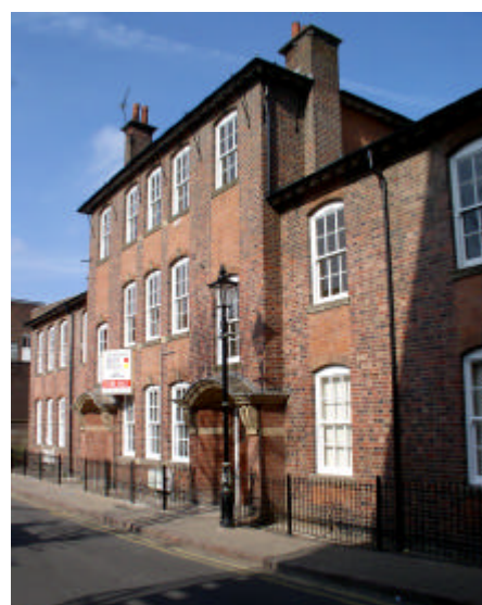
The recent conversion of 8 Mill Hill Lane, into flats, with re-instated timber sash windows.
