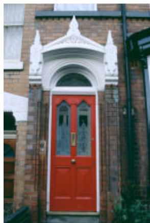
An original two panelled door with etched glass windows - Severn Street.
