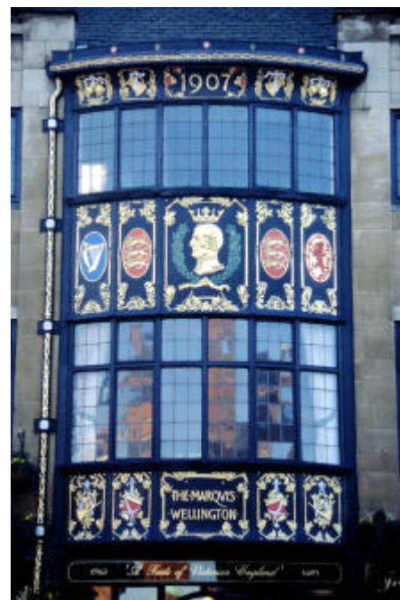
Decorative leadwork to the Marquis Wellington pub, London Road.
