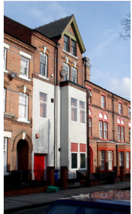
Highfield Street: Inappropriate materials can have a major detrimental affect on the appearance of an area.
