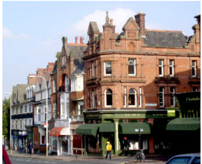
A fine group of original shopfronts at the corner of Highfield Street and London Road.
