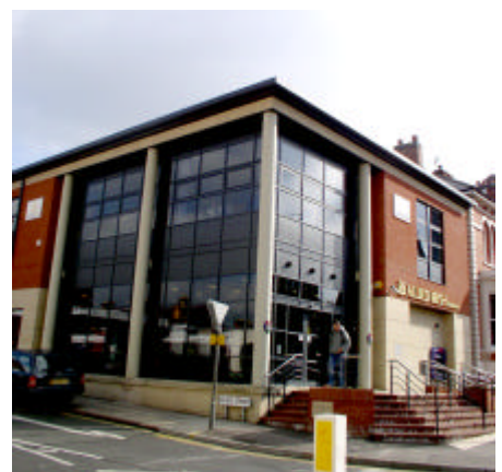
The well-detailed new office development at 1-3 Saxby Street uses quality materials and respects the height and scale of adjoining properties.
