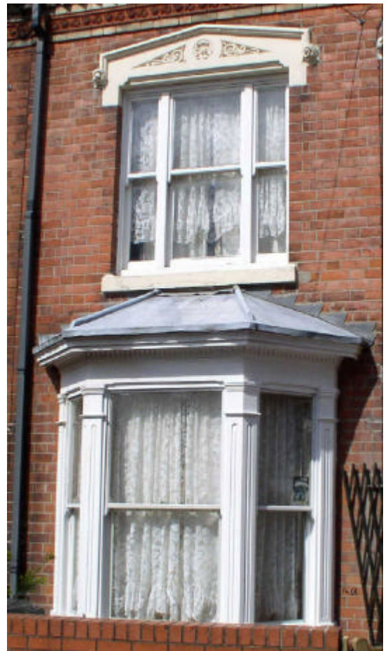
Attractive timber bays and finely-detailed traditional sash windows are one of the most important architectural features of South Highfields and make a major contribution to the architectural character of the area.
