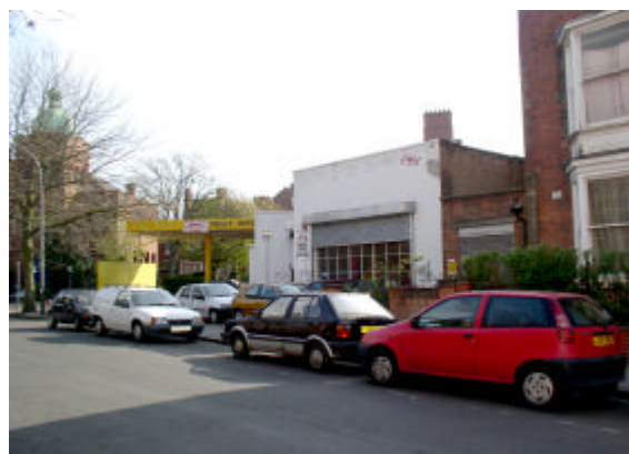
The single storey property at the corner of Tichborne Street and Highfield Street is detrimental to the area.
