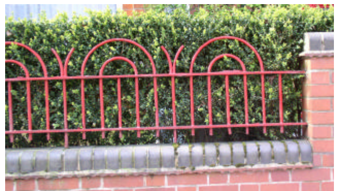
Simple, well-designed bow-top railings, Severn Street.
