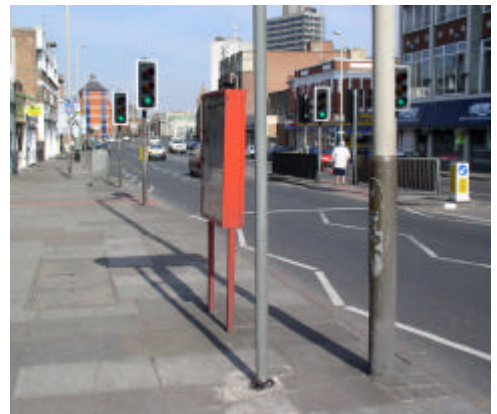
Excessive posts and signs give a cluttered appearance along London Road.
