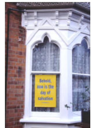
'Gothic' style wooden bay in Severn Street.
