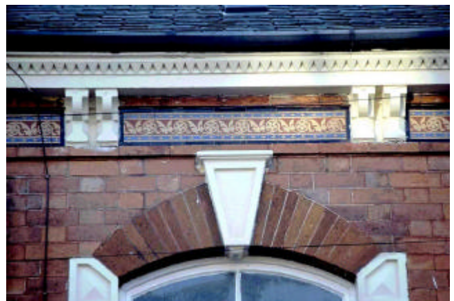
An example of the finely decorated cornice detail with encaustic tile border typical of the South Highfields area.
