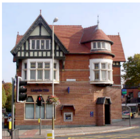
The original ground floor elevations to 1 St. Albans Road were lost in the 1950s, (see historical image on p7).
