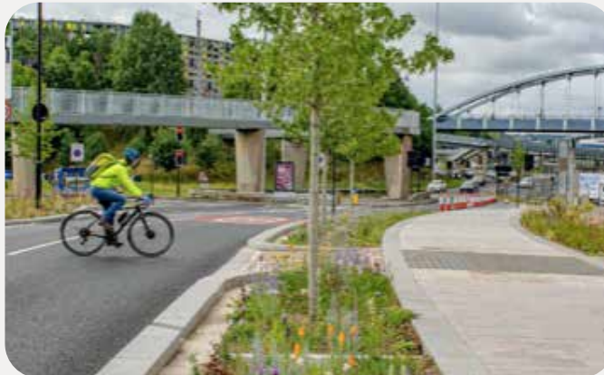
Figure 31. Street Swales Take Surface Run Off from the Carriageway & Provide Landscaping & Tree Planting, Sheffield
