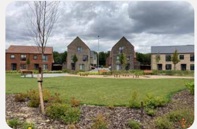
Figure 95. Pocket park fronted by 'set piece' frontage, Cambridge
