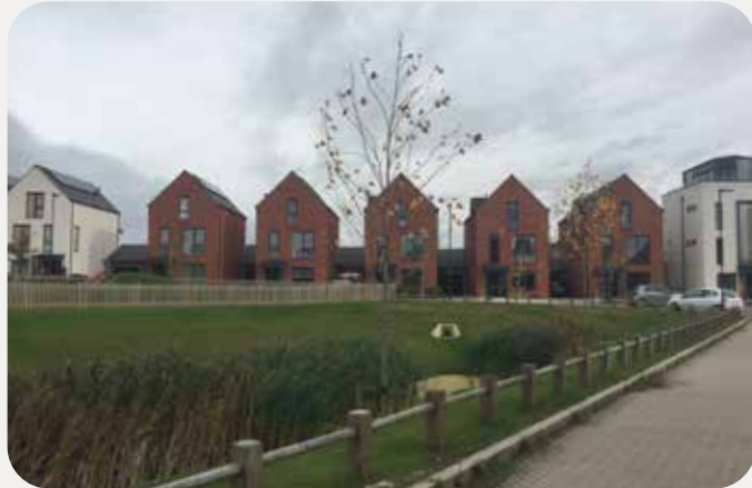
Figure 46. Same House Type to Create a Distinctive Edge to a Green Space, Derby
