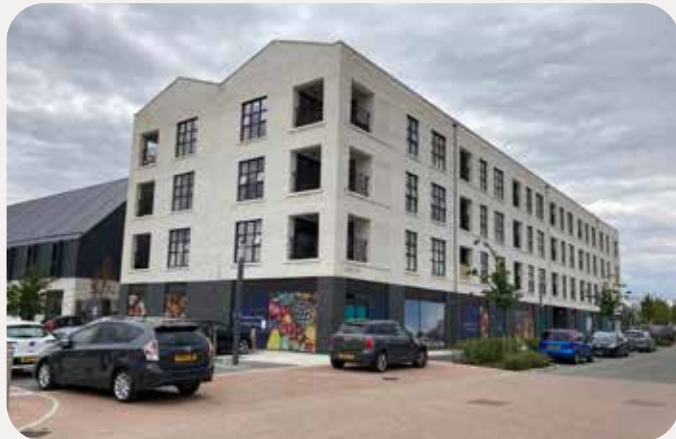
Figure 61. Distinctive block of flats with store below, Marleigh, Cambridge
