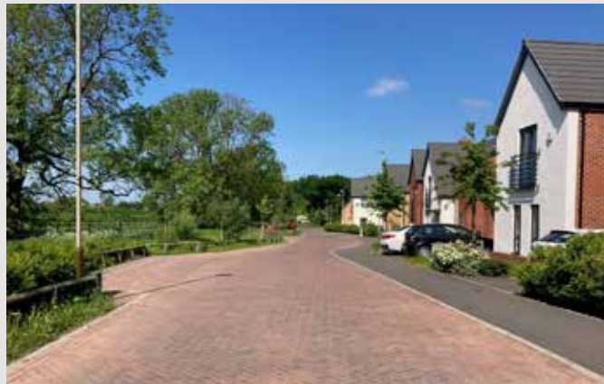
Figure 109. A Green Edge Street Widened to Provide an Informal Edge for Car Parking
