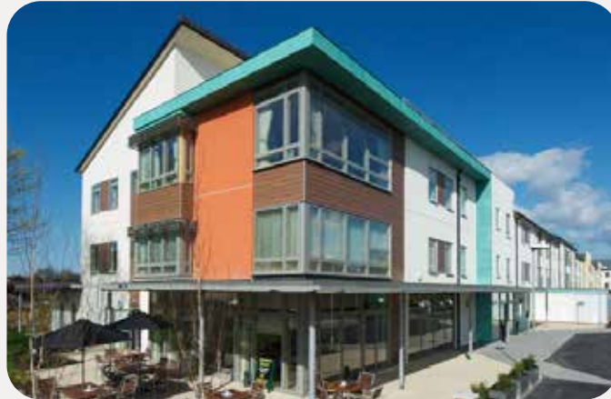
Figure 59. Building Designed with a Prominent Corner, Providing a Unique Local Marker & Legibility
