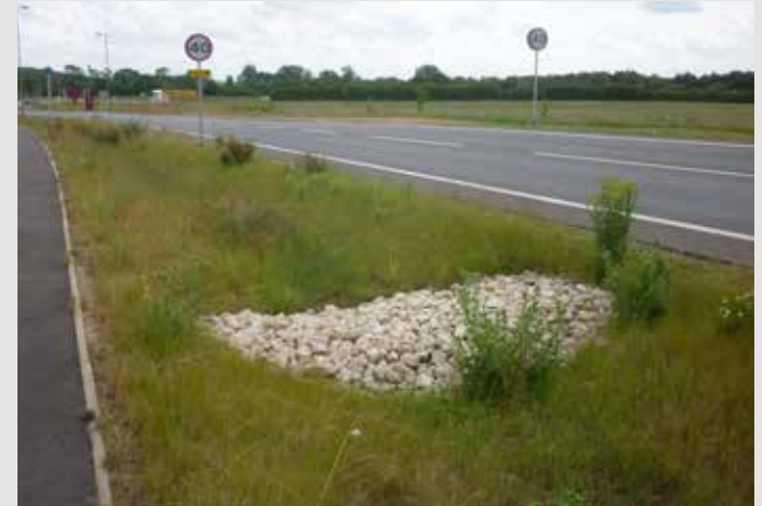
Figure 117. Simple Check Dam with a shallow swale, Oxfordshire
