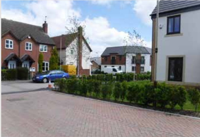
Figure 113. Permeable Paving, Getliffe Road, Ashton Green Phase 1
