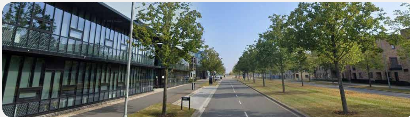
Figure 44. Employment & Enterprise Zone, Alconbury – Strong Building Frontages & Legible Entrances to Main Street
