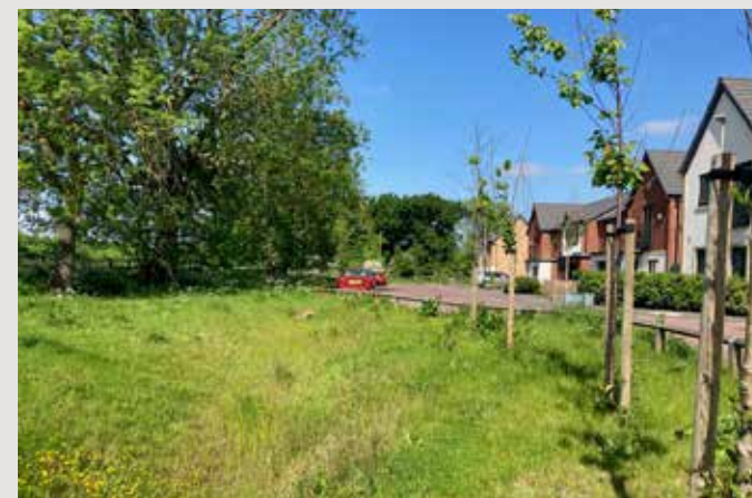
Figure 110. Street draining at grade into adjacent swale, open space Ashton Green
