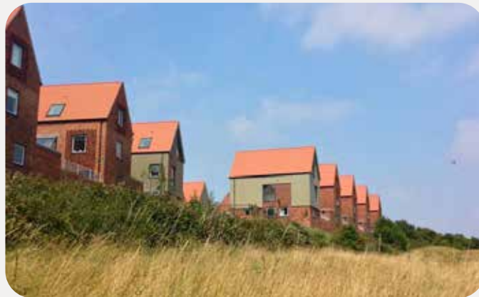
Figure 43. High Quality Homes to a Prominent Frontage, Horsted Park, Kent
