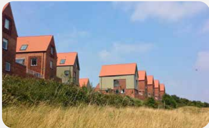
Figure 39. High Quality Homes to a Prominent Frontage, Horsted Park, Kent
