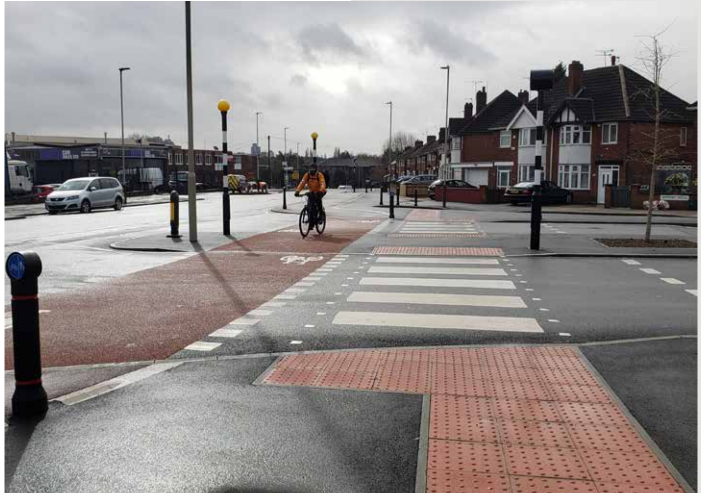
Figure 107. Full Set Back, Marked Priority (bent-out) Crossing, Parker Drive, Leicester
