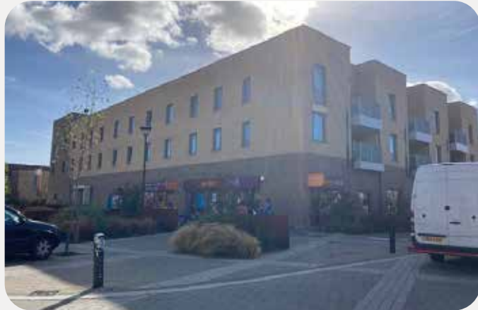
Figure 58. A Sainsbury's Store with Flats Above, Cambridge
