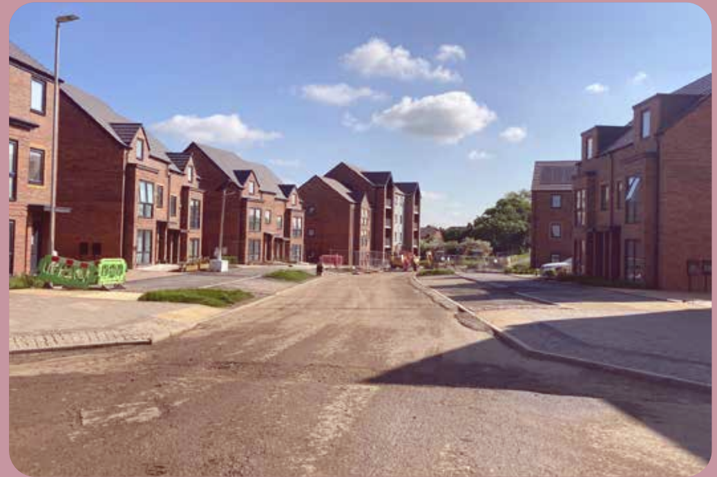
Figure 124. Bevan Road Code D (Under Construction)
