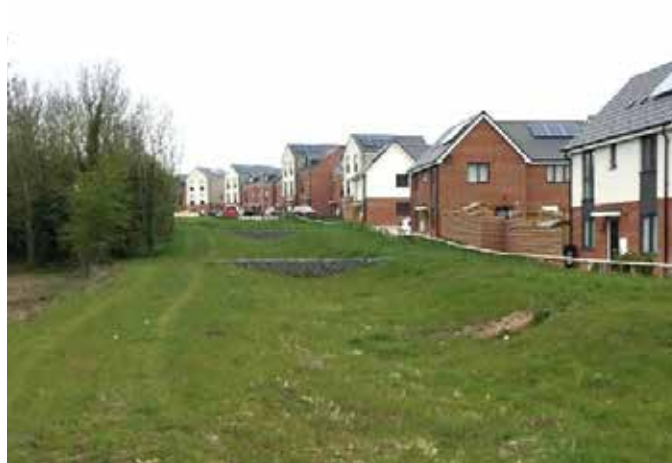
Figure 115. Gabion Crossing of Swale, St. Mary's Allotments, Leicester
