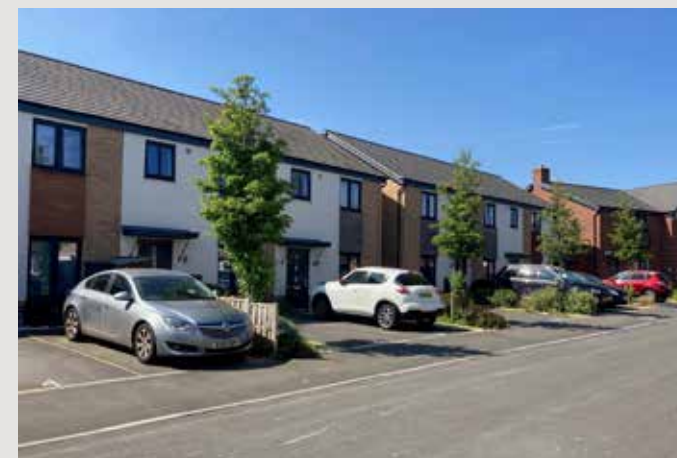
Figure 131. Tree Planting Reducing the Visual Impact of Front On Plot Car Parking, Ashton Green Phase 1
