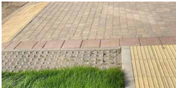
Figure 104. Place-Making Junctions Along Bevan Road (Under Construction)
