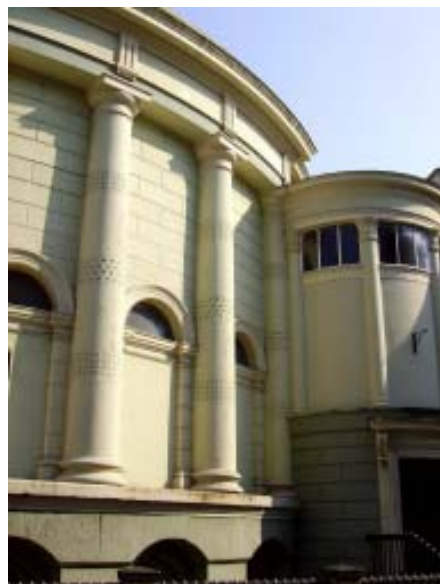
A detail of the stuccoed Roman Tuscan columns to the Adult Education College, Belvoir Street.
