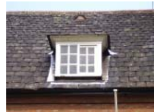
Swithland slate to the roof of 20 Millstone Lane
