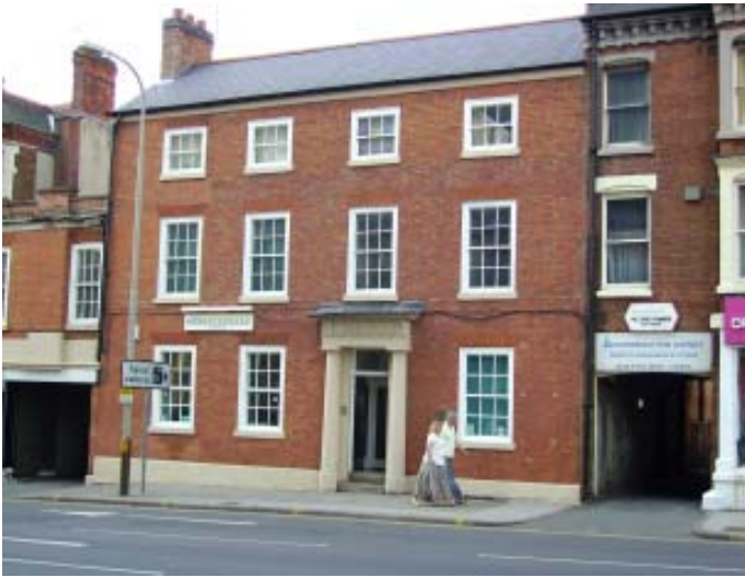
The three storey former Georgian dwellinghouse at 11 Welford Road is listed Grade II; the fine Doric style doorcase is set off centre.
