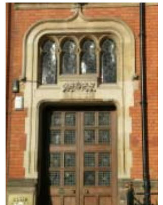
Stone gothic detailing to fanlight and doors at 9 Welford Place.
