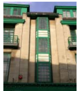
Fenwicks Belvoir Street: steel windows and Vitriolite panels
