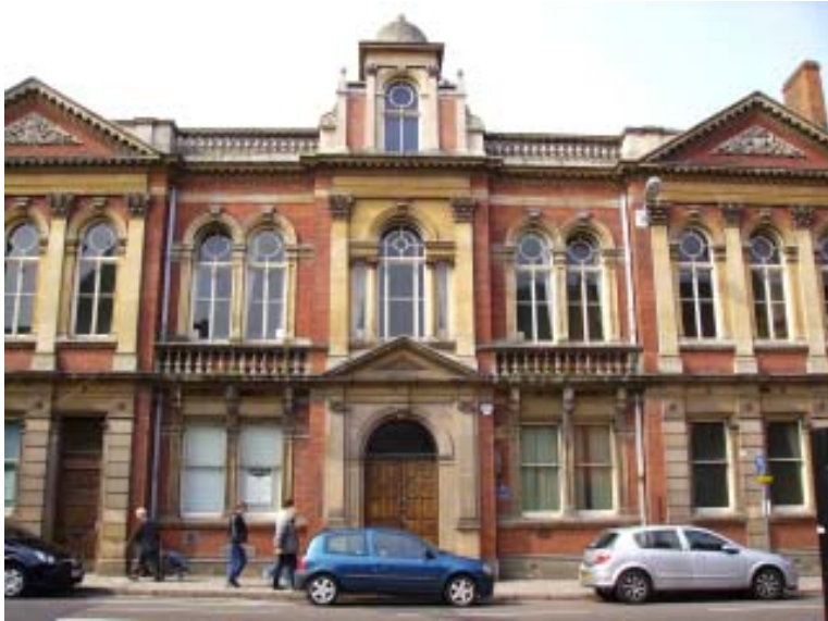
The former Registry Office, Pocklington's Walk, designed by Redfern and Sawday as Poor Law Offices in 1883. Built in the Jacobean style, it features a fine Venetian first floor window above the central entrance doors.
