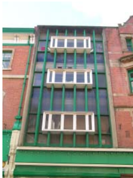
This particularly interesting Modernist style infill to the Fenwicks store in Bowling Street dates from the 1950s.
