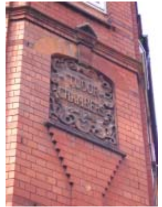
Moulded brickwork to the corner of 25 Millstone Lane.
