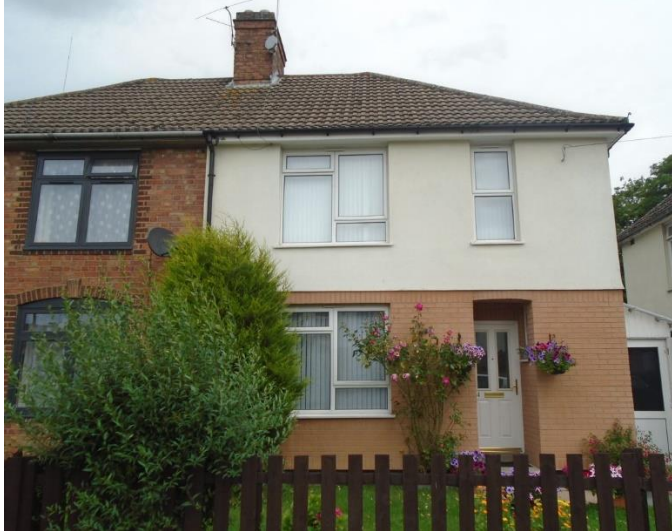
EWI finished with half brick slip and half plain smooth render above.
