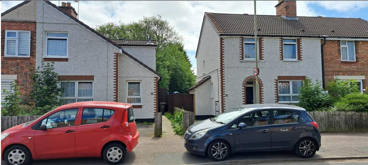
Two examples of EWI finished in pebble dash render with carefully positioned brick slips to retain character/detailing of the area
