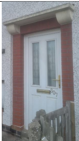
Brick slips for door surround
