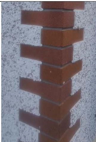
Detail of pebble dash and brick slip finish
