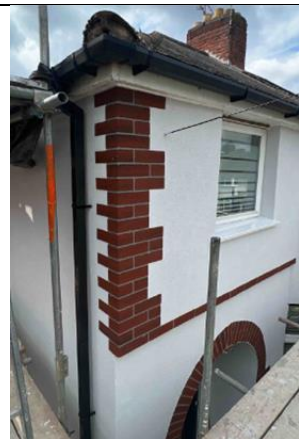
Brick slips for corner detailing
