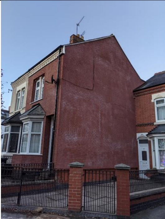
EWI finished with brick slips in a mixed hue finish with eaves detailing replicated.
