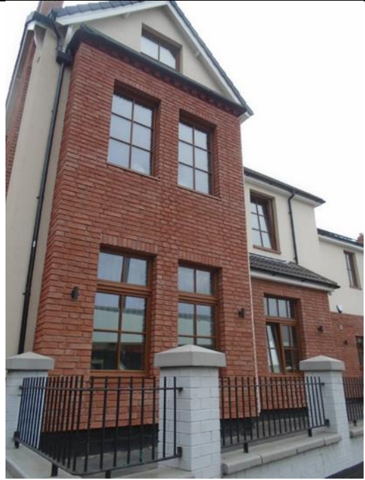
EWI finished with a balanced contrast with brick slips and plain smooth render.
