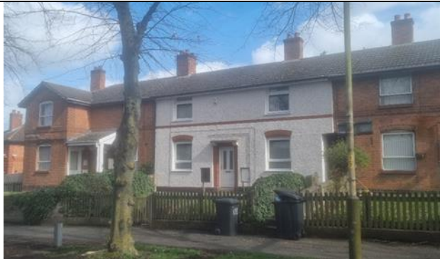
Brick slips for door surround, central banding and lintels
