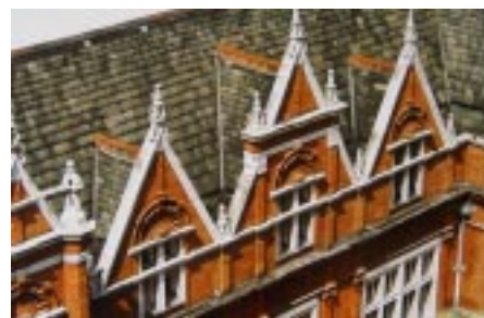
Swithland slate to roof of 17 Horsefair Street.
