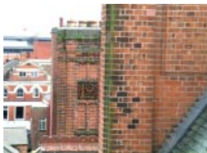
Moulded brick detailing to Town Hall chimney stacks.
