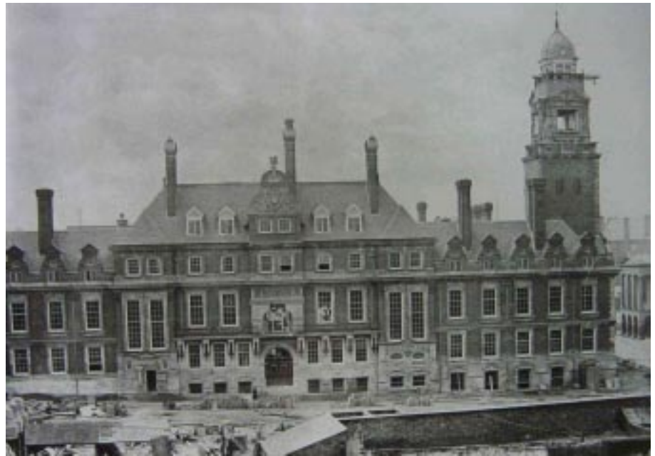
The Town Hall nearing completion. Note the Cattle Market buildings in the foreground.
