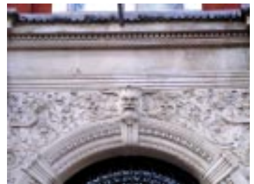
Carved stone detailing at 17 Horsefair Street.
