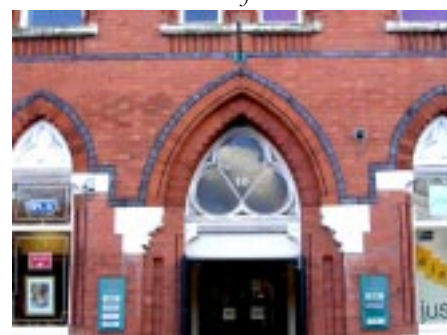
At 10 Bishop Street a variety of materials was used to create the 'Gothic' style: Leicester red brick; 'stringcourses' of blue brick; stone corbelling and a fanlight of stone and cast iron.
