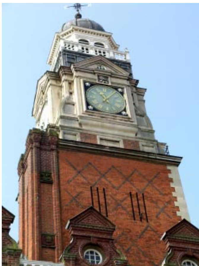
The Town Hall Clock Tower is a major landmark within the Conservation Area. It is rich in architectural ornamentation including striking blue diaper brickwork, Ketton stonework, and an octagonal timber lantern with balustrade, all crowned by a lead covered cupola.
