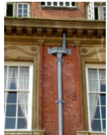
Moulded and dated lead rainwater hopper and down pipe, Town Hall.
