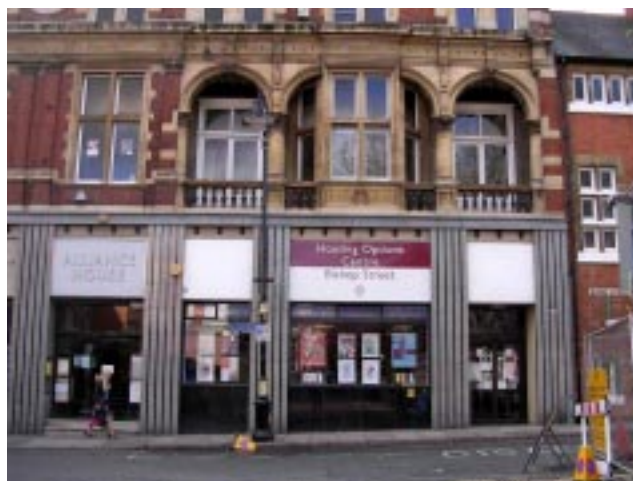
Shopfront to Alliance House, 6 Bishop Street.
