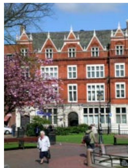
The façade of the former Sun Alliance offices dates from 1891.
