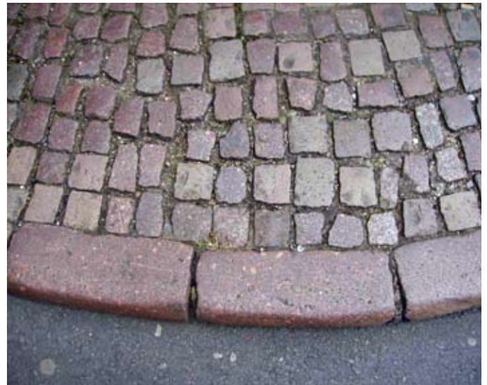
Mountsorrel granite setts and kerbs are an important local feature within the Conservation Area.
