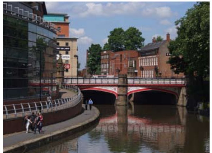
West Bridge designed by E. C. Mawby the Borough Engineer in 1890.
