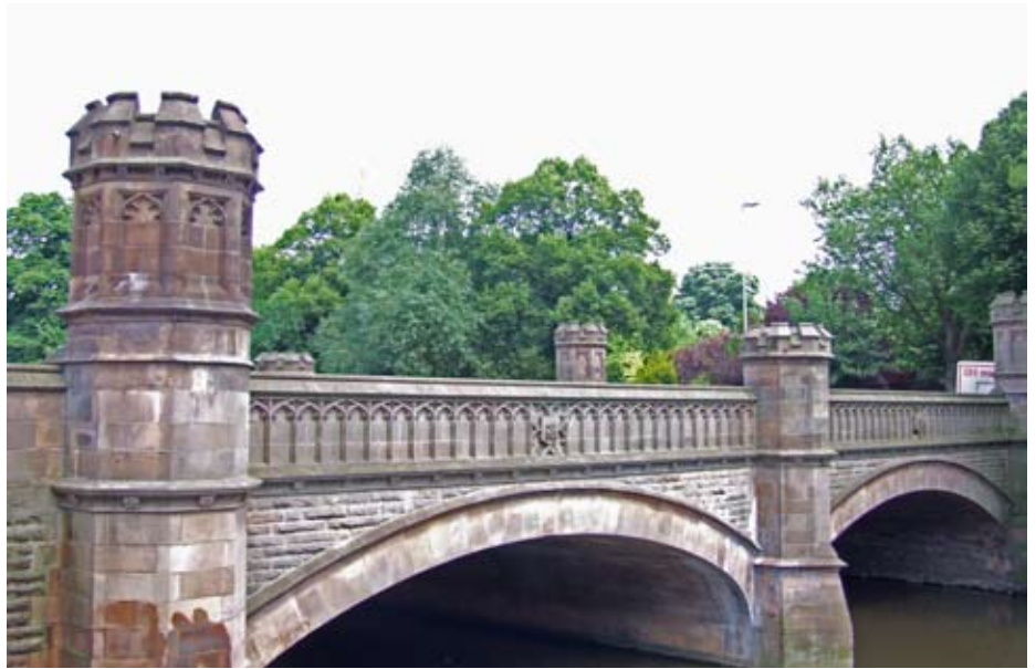
The Newarke Bridge completed in 1898 and constructed using large ashlar blocks.
