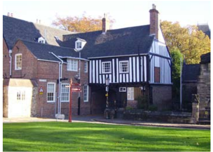
The rear elevation of the Castle Gatehouse seen from Castle Green.
