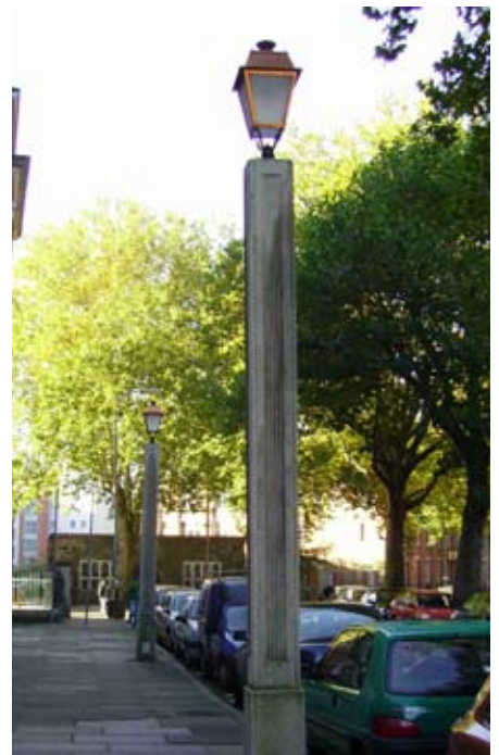
Above: These two unique square section lamp posts date from the 1930s and were installed at the time that the Hawthorn Building was constructed. The copper lanterns are an unfortunate recent change. The original square shaped lamps were designed to complement the design of the columns as is evident from the top image.
