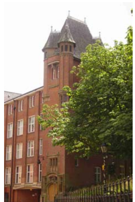
The tower to the former Stretton's Hosiery factory, Castle Street.
