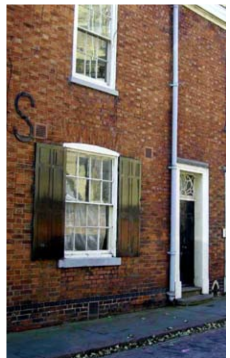
External wooden shutters to cottage in Castle Street.
