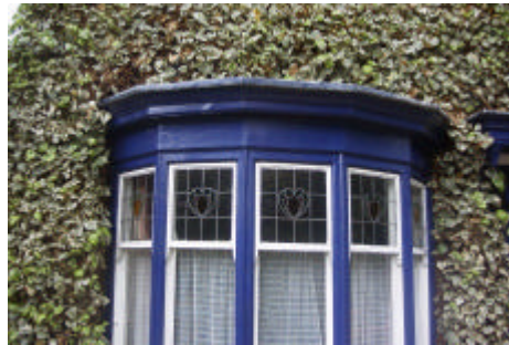
Semi-circular bay window - St. Saviour's Road
