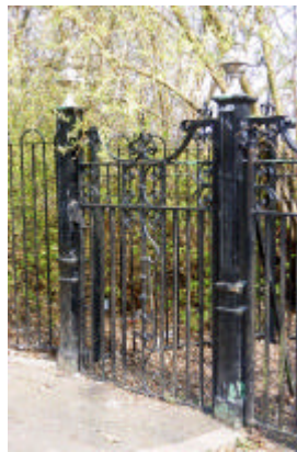
Cast iron gate and piers to the park boundary.
