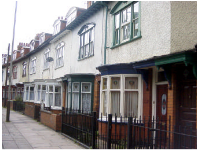
The gently curving terrace between 220 and 248 St. Saviour's Road has unusual curved timber pediments to first floor windows and interesting curved wooden dormers above.
