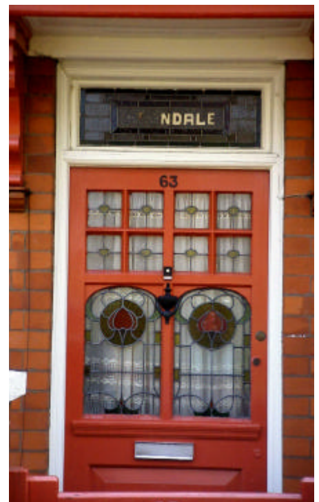
One of the many original front doors typical of the conservation area. This one features a complete set of fine leaded and stained glass.
