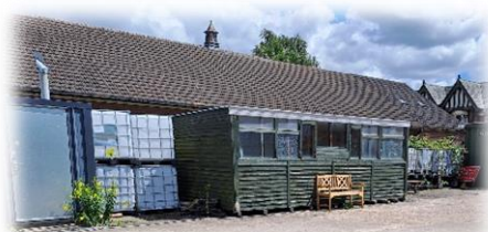
Evington Parks rainwater collection.
