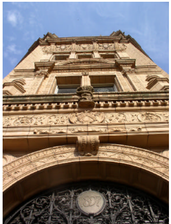
ABOVE and TOP: No expense was spared in the construction of Alexandra House. Great use was made of terracotta, polished Norwegian larvikite, (a type of granite) and etched glass in cast iron frames in the sumptuous decoration.
