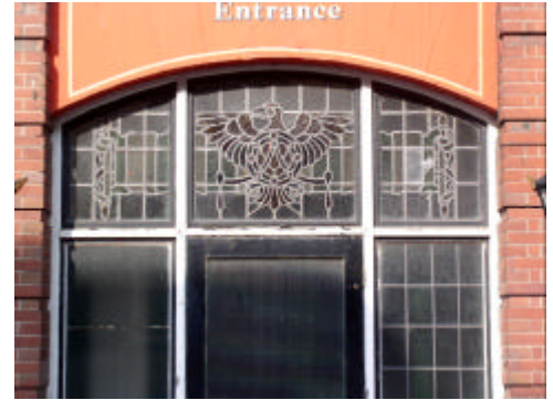
Leaded window with eagle motif to side entrance of former Spread Eagle Public House, corner of Charles Street and Church Street.
