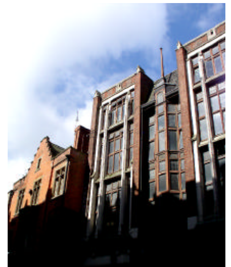
78-80 Rutland Street is very unusual and is eclectic in style with Gothic, American and other architectural influences.
