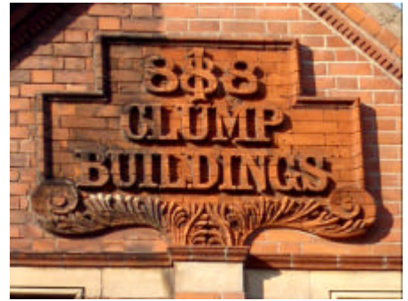
Moulded brick at 8-32 Humberstone Gate.
