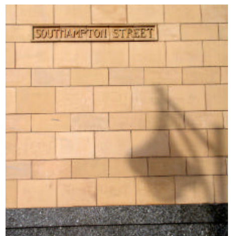
Alexandra House: The incorporation of the street nameplate into the terracotta tiling shows great attention to detail.
