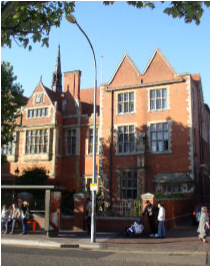
Clarence House (now Age Concern), was designed by Edward Burgess as a school and was opened in 1879.
