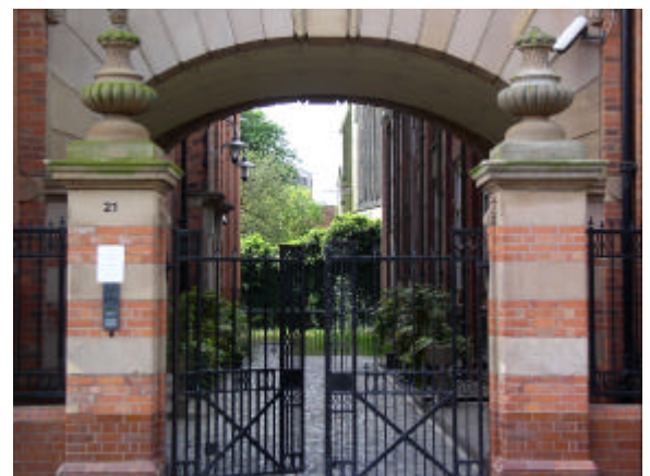
The baroque gateway to the former Rowley's factory Queen Street, gives a surprise view towards the west end of St. George's Church and Churchyard.
