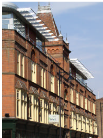
The Exchange Building, Rutland Street, was designed by Stockdale and Harrison of Leicester and dates from 1888.
