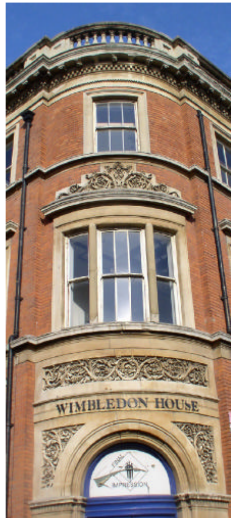
Wimbledon House at the corner of Wimbledon Street and Southampton Street makes the most of its prominent corner location with a highly detailed ornate entrance designed in the Italian style.
