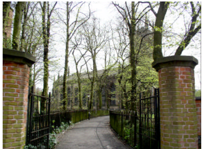
St. George's Churchyard: the bow-top railings and entrance gates were manufactured locally by S. Wright and Co.
