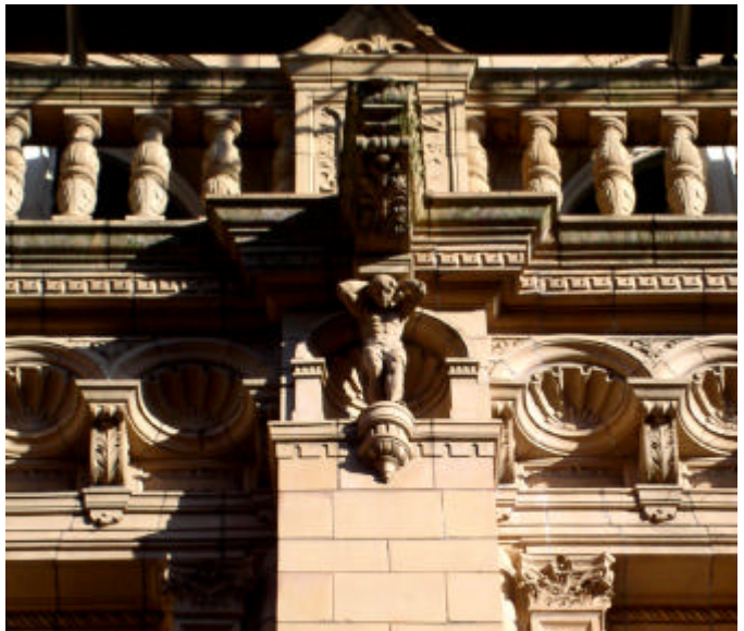
Alexandra House: one the ten figures of Atlantes holding up the cornice brackets.
