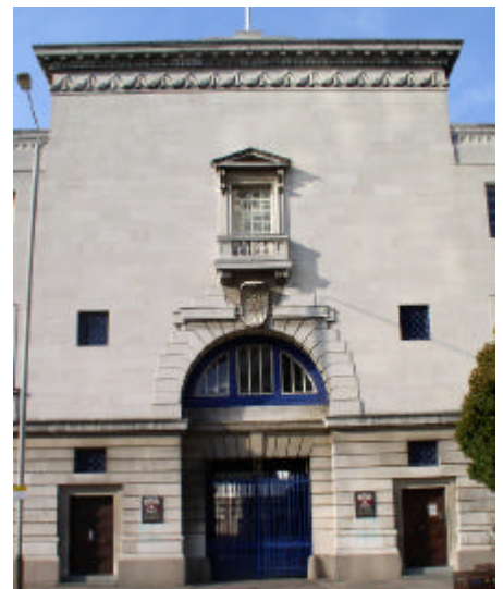
Area 3: Former Central Police Station, Charles Street, of 1933 designed by architect Noel Hill.
