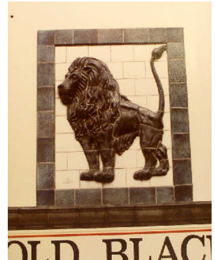
The Black Lion Public House has two dellt tiled panels showing a striking lion modelled in bas-relief. Regrettably, the black tiled figures have now been covered in gold paint.
