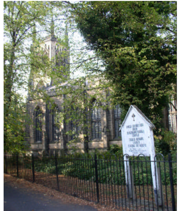
St. George's Church is one of the few buildings in the Conservation Area constructed from stone; it also has cast iron window tracery.
