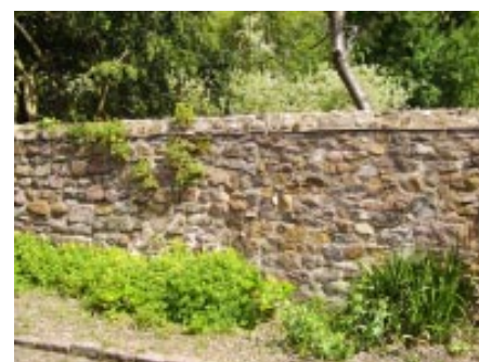
Boundary wall to Humberstone Manor.
