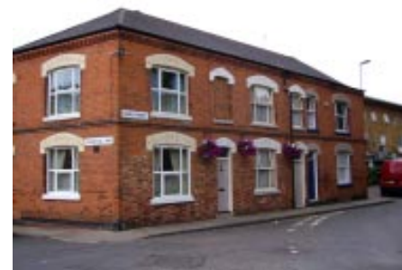
Top: Victorian terraced properties at 79-83 Main Street showing a previous conversion to shop use and above, their more recent successful restoration back to residential use.
