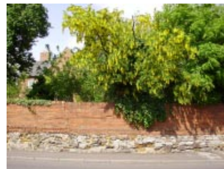
A combination of brick and random stone used for construction of boundary walls is one of the key distinctive elements used within the conservation area.
