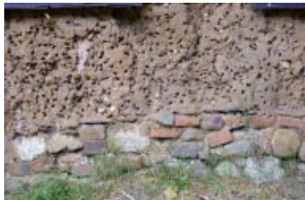
Section of mud wall, St. Mary's Churchyard
