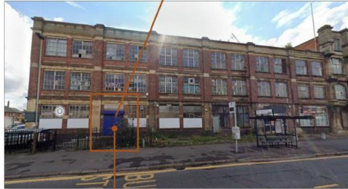
CUSTOMER ACCESS DOOR
