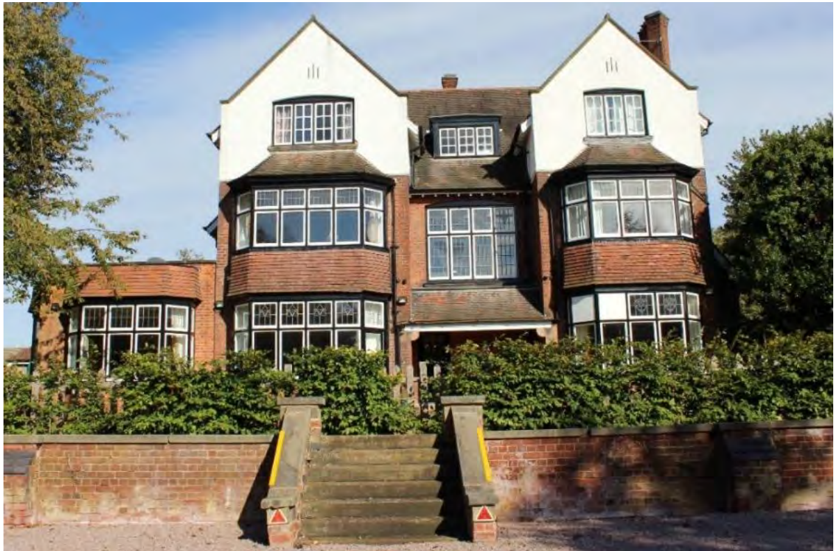
The South frontage of Latimer House overlooks the entry onto the Attenborough Arboretum. The building is of notable architectural value.
