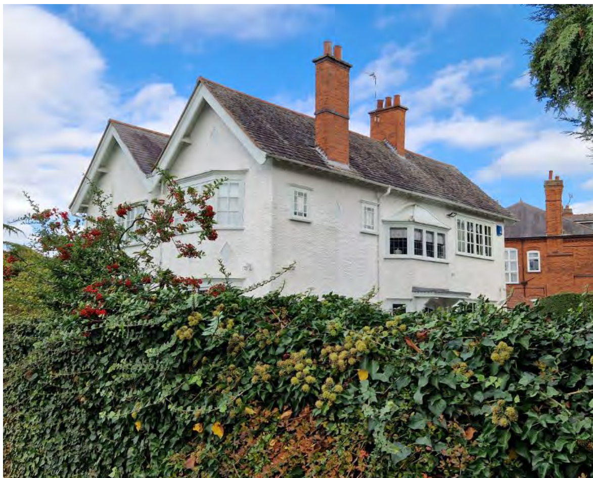
185 Ratcliffe Road. A Swithland Slate roof is visible on the right roof ridge.
