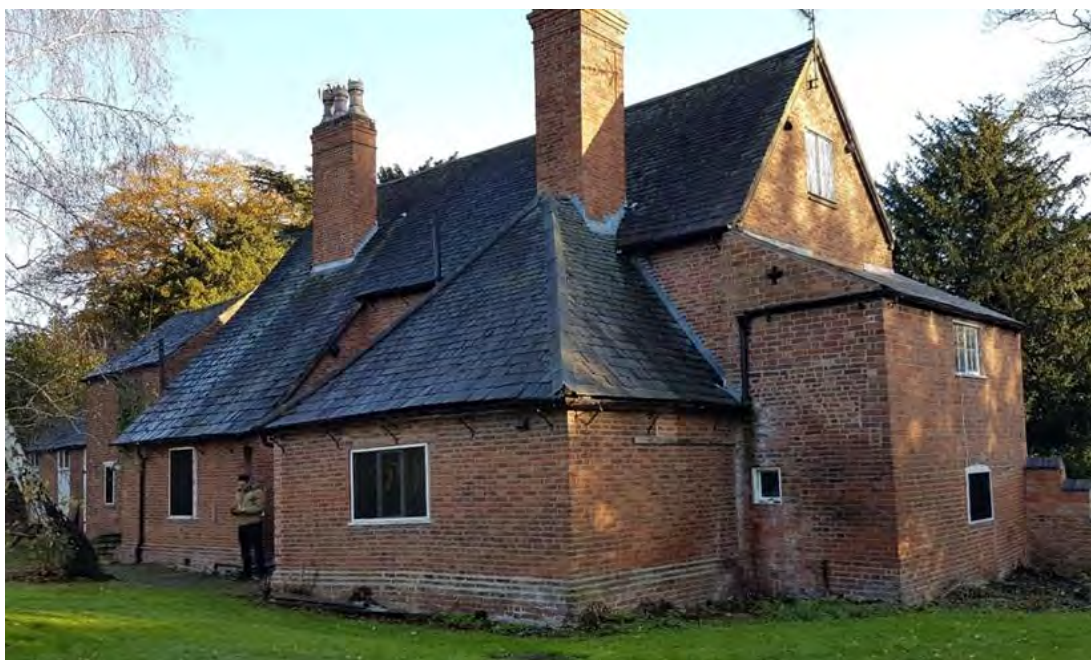
The Grove is an architecturally restrained farmhouse, with steeply pitched Swithland slate roofs and mixed red brick elevations.
