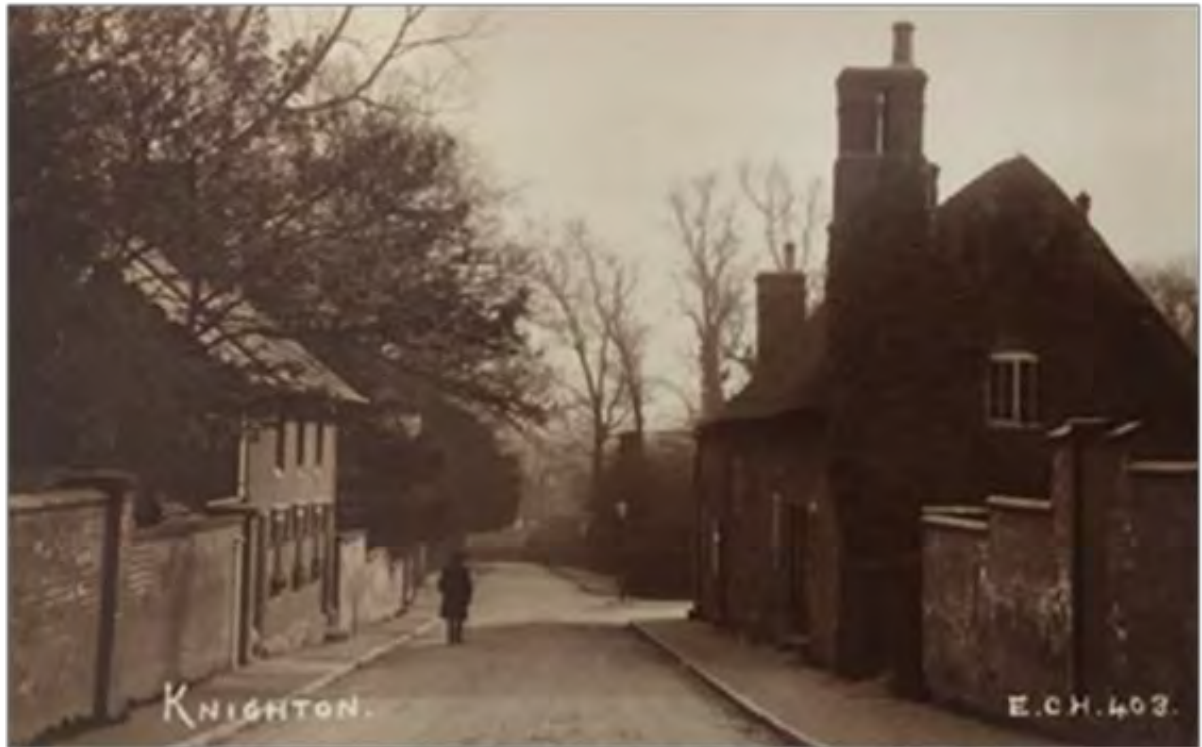
View along Knighton Road onto Church Lane, with the two brick dwellings since demolished.
