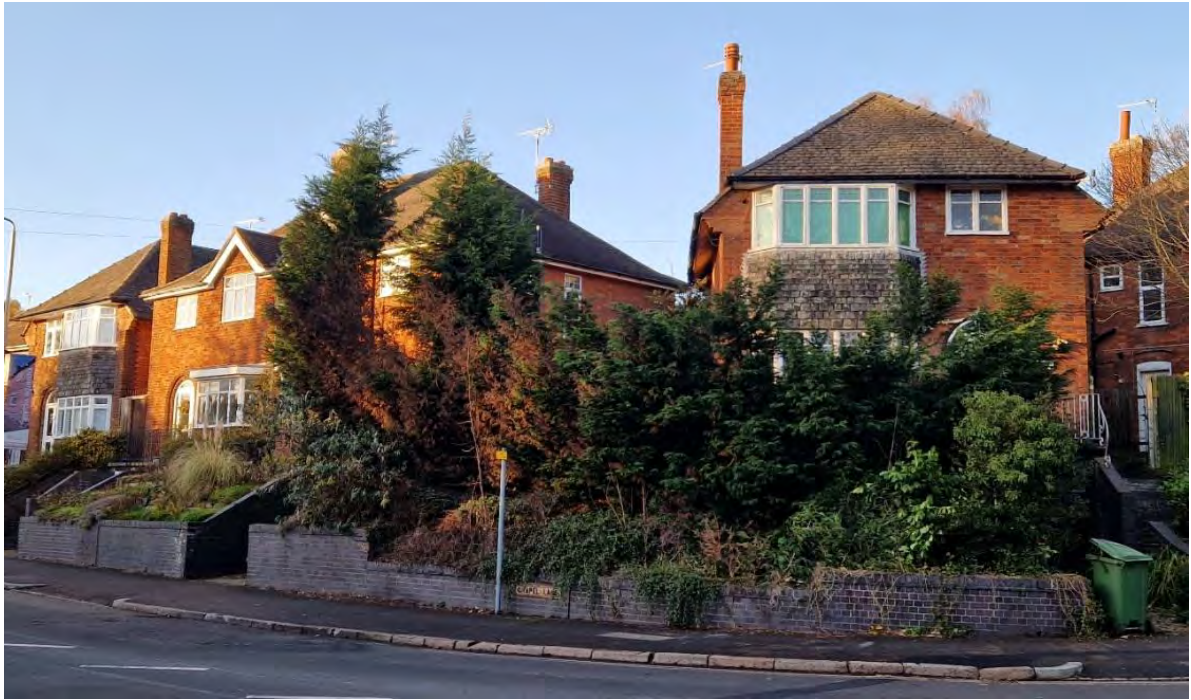
The 20th century dwelling at 44-48 Chapel Lane. 44 uses Swithland slate on the roof and in the shallow canted bay.
