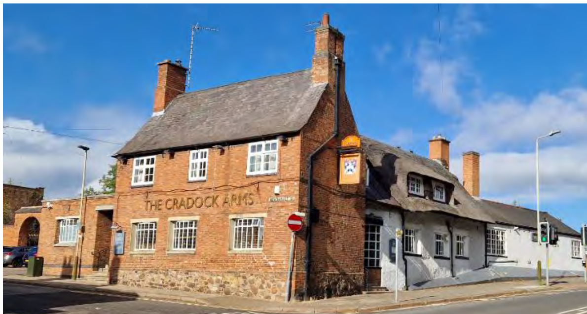
The Cradock Arms is one of the oldest buildings in the conservation area
