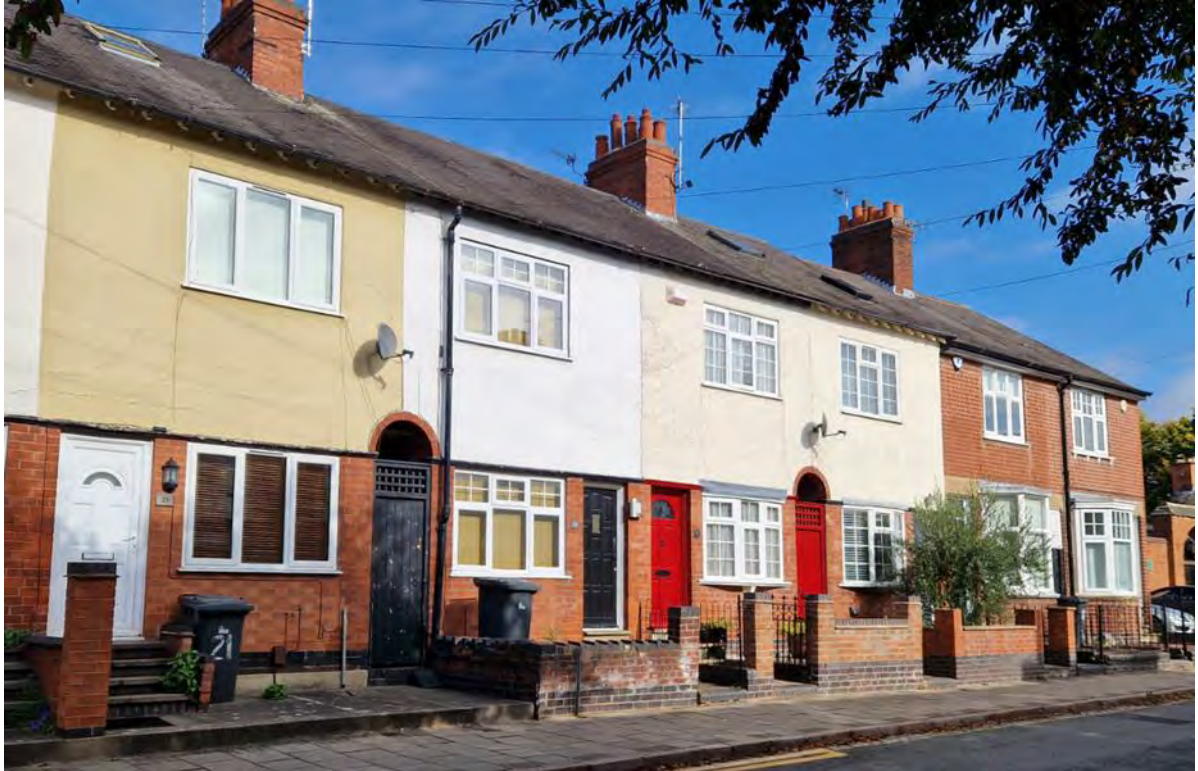
Terraced dwellings at 11-21 Newmarket Street
