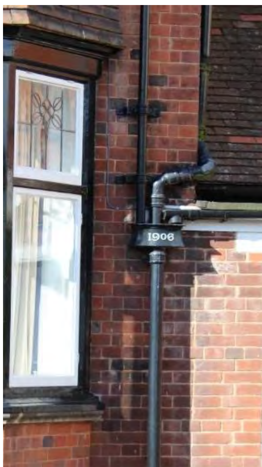
Left: The date stamped cast iron hopper at Latimer House.
