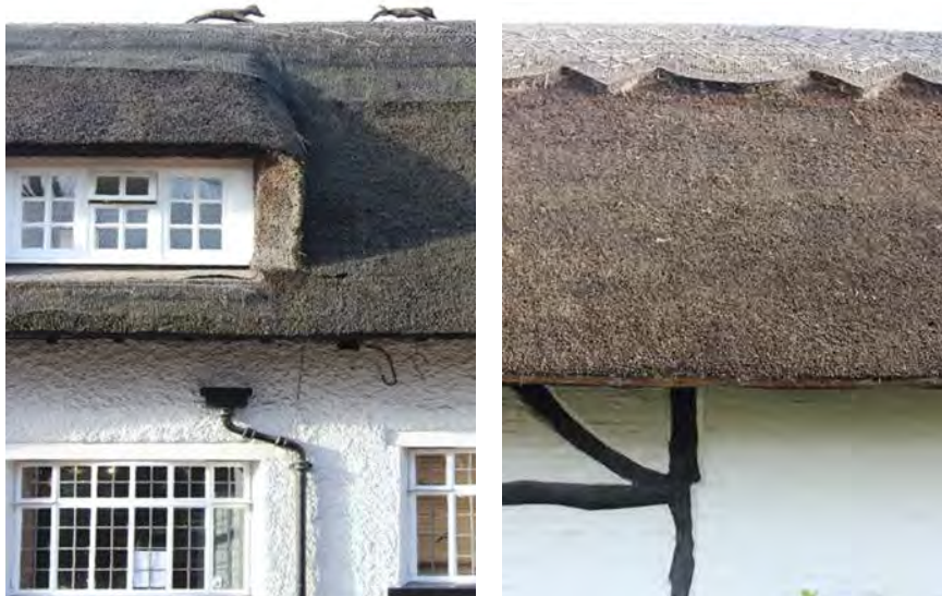
The thatched roof of the Grade II Listed Oram Cottage, with decorative pattern to ridge.
