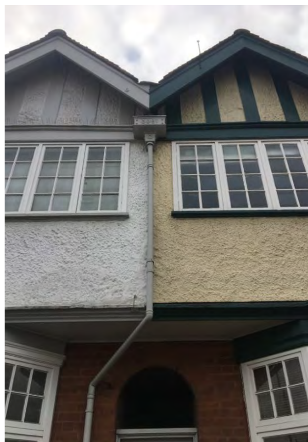
Right: Decorative timber gables and bargeboards on jettied upper floors evoke a vernacular tradition on Knighton Road
