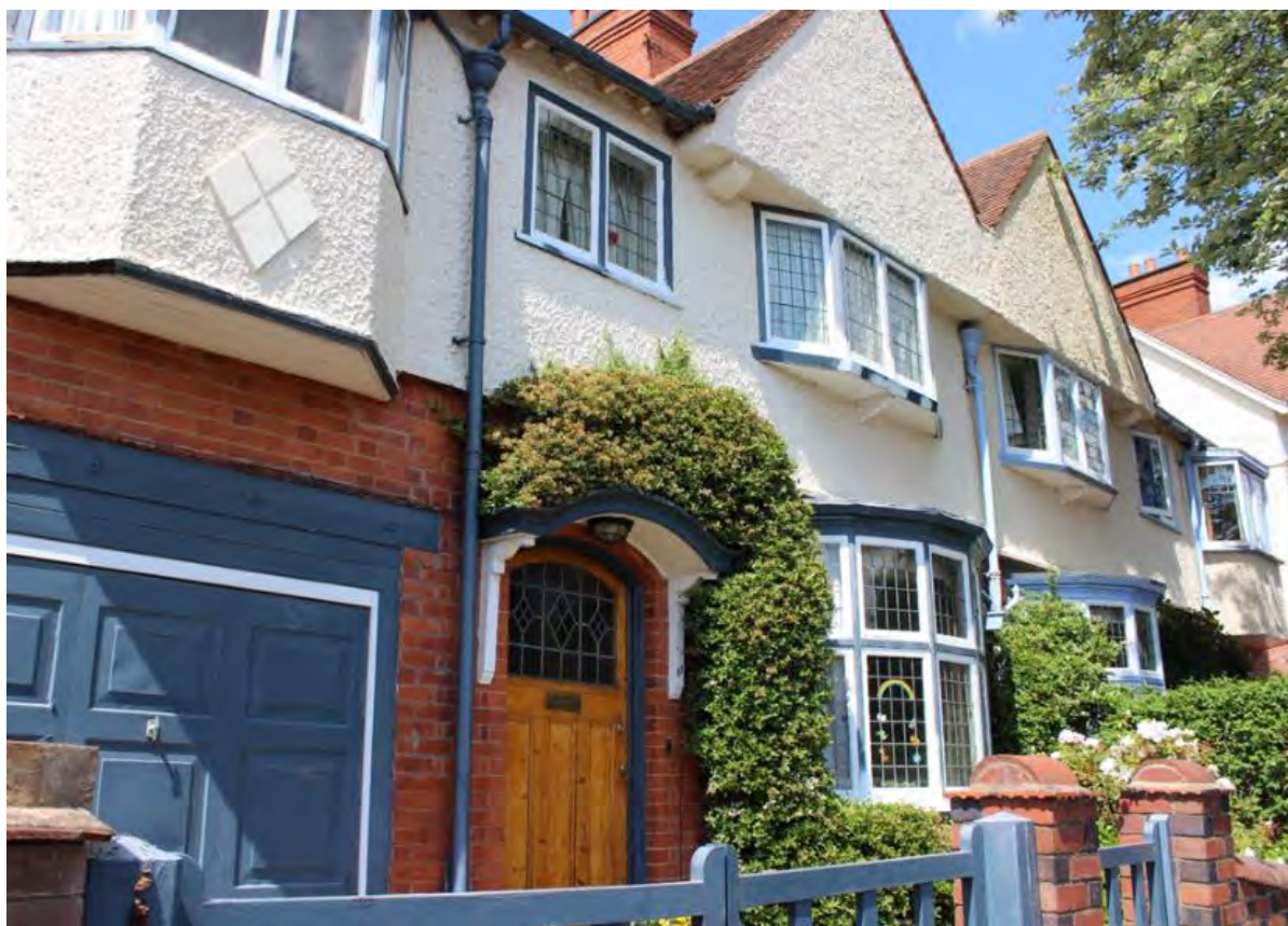
The frontage at 7-9 Carisbrooke Road features a multiplicity of elegant architectural features that animate the local streetscene
