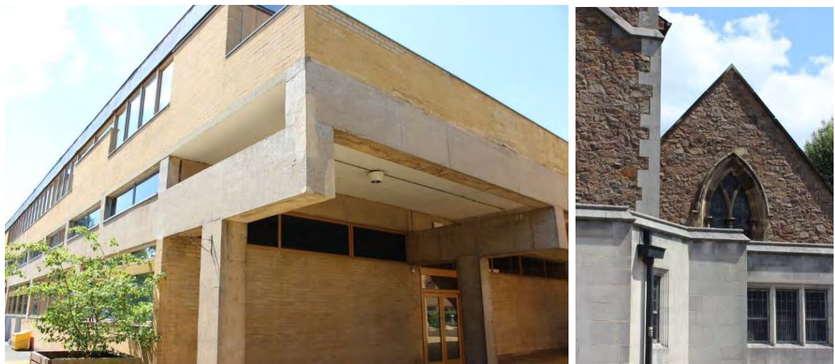
Left: College Court is characterized by a mix of facing materials, including buff brickwork, timber and lead cladding; together with its exposed concrete elements.
