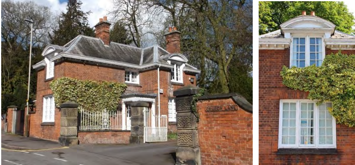
The lodge, wall and gates are all curtilage listed and form an attractive group
