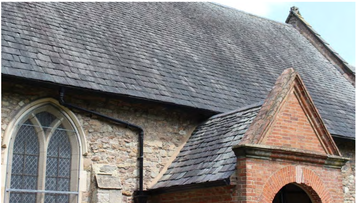
The southern roof of St Peter's Church has a large expanse of prominent Swithland Slates laid in diminishing courses
