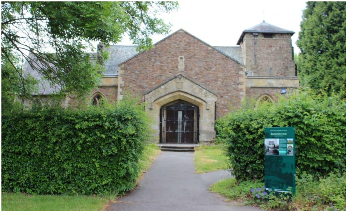
The imposing north entrance to St Peters Church dates to the 1930s and was part of an unfinished proposal to re-orientate the church.
