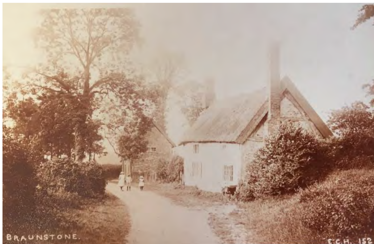
Photo of now demolished house on Braunstone Lane
