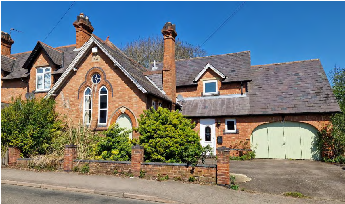
The frontage of the former National School is the single most architecturally embellished element of the structure, with stone dressing, a commemorative carving, and a moulded bargeboard.
