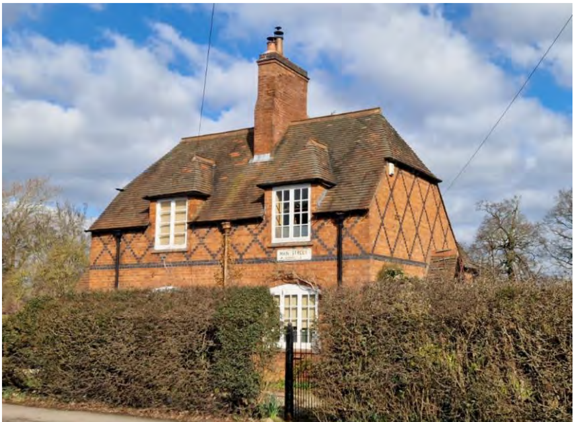
1 & 2 Main Street. The diaper brickwork at comprehensively defines the upper portion of the dwellings' frontage
