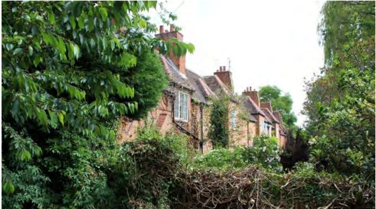
Cressida Place cottages are obscured by mature planting and complimentary soft landscaping, creating a picturesque townscape.
