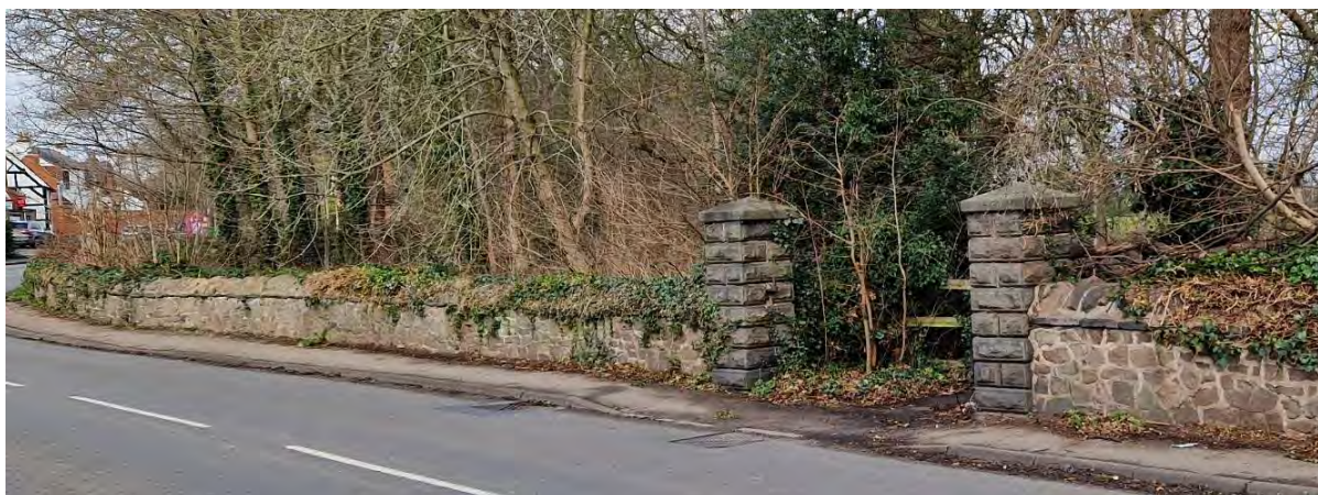
The low rubble stone wall to Church Field is a unique feature within the Conservation Area. The rusticated gate piers appear to be a later feature and are of a non-local granite.
