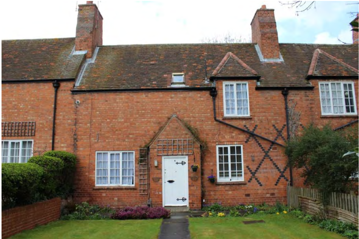
The front elevation of each property is of slightly different design featuring diaper brickwork, dormers, shallow porches, timber casements and moulded chimneystacks.
