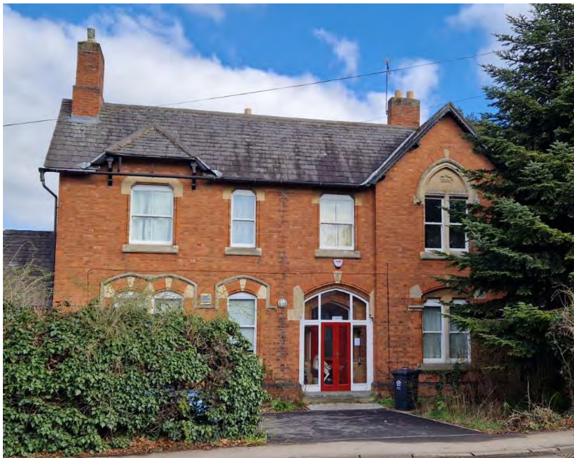
The frontage of St Peter's Vicarage is framed and partially obscured by mature conifers. It features stone dressings in the form of carved hood moulds and an engraved date.
