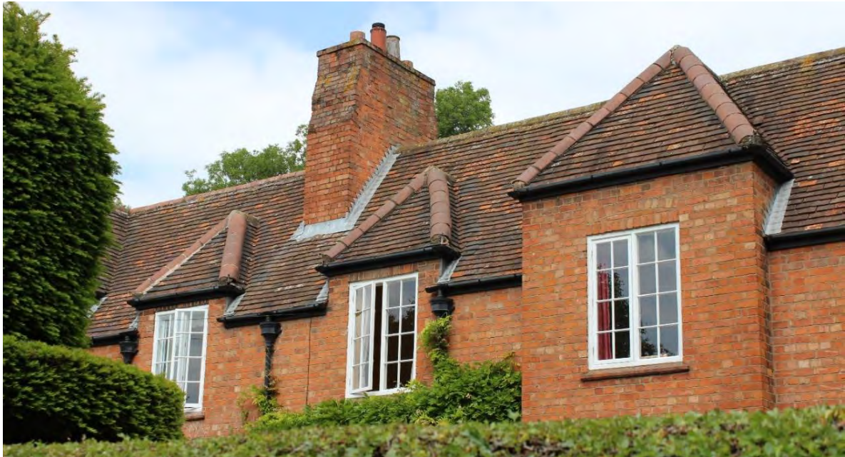
Roof detail at Cressida Place
