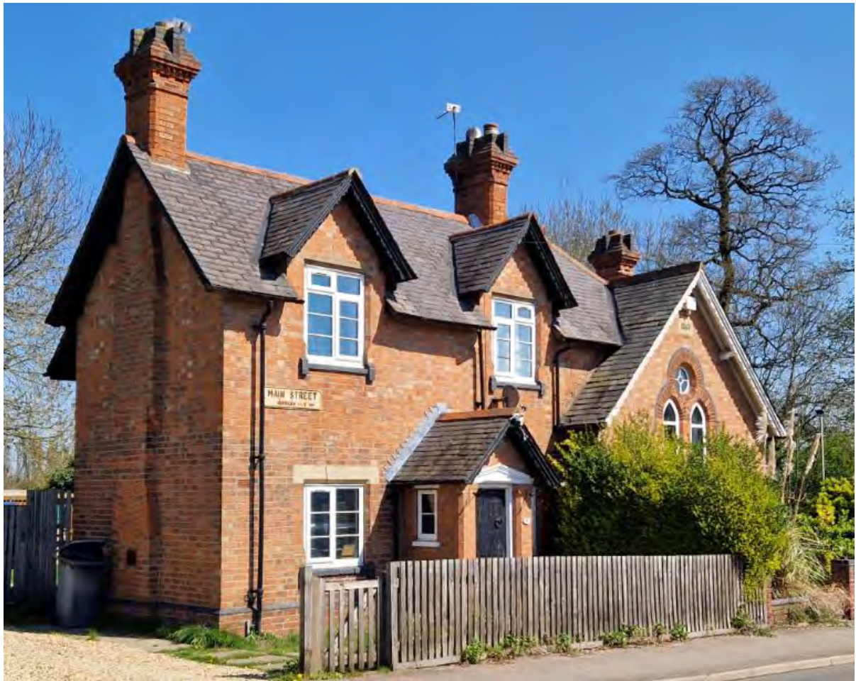
Former Schoolmasters House with gabled dormers above
