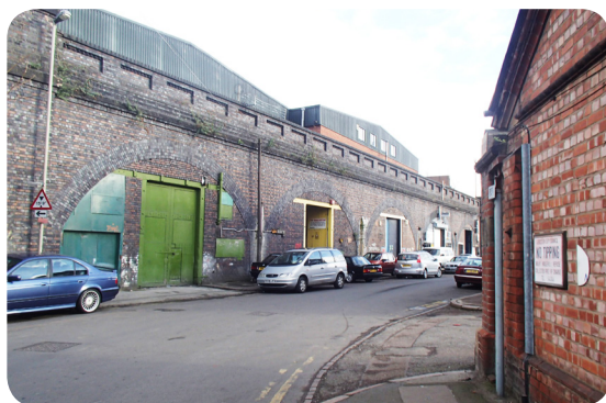
Viaduct arches on Jarvis Street
