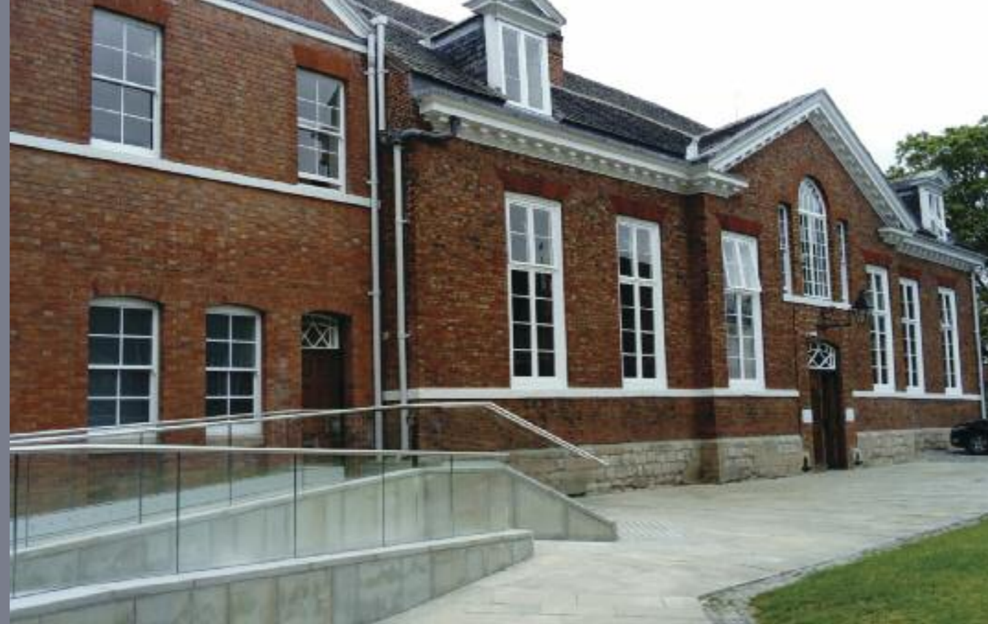
The Castle following renovation work
