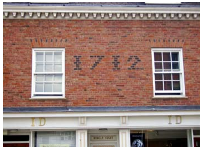
Eighteenth century brickwork at 21-23 Highcross Street.
