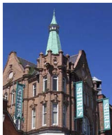
Terracotta and copper materials used at 10 East Gates
