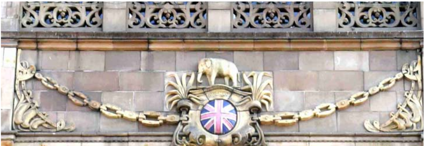
Moulded faience decoration at second floor window height of 76-88 High Street, (former Coronation Buildings).
