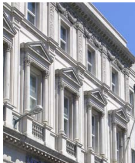
Lloyds TSB bank premises at 7 High Street, constructed from Portland stone in the Classical style.
