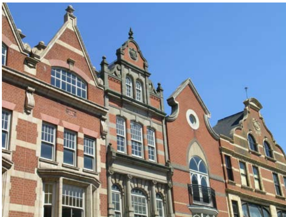
Skyline architectural details to the north side of High Street..
