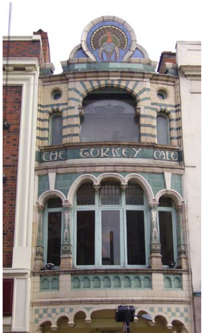
The Turkey Café was built to the designs of Arthur Wakerley in 1901. The exotic Turkish/Persian style moulded and glazed terracotta was made at the Doulton Pottery in Lambeth.
