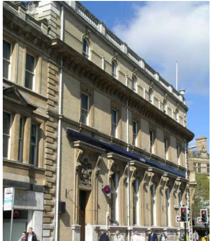
Number 1 Granby Street was designed in the classical revival style. The stone work is particularly fine with a strong horizontal rhythm created by the large stone console brackets and the stone cornices at first and second floor levels.
