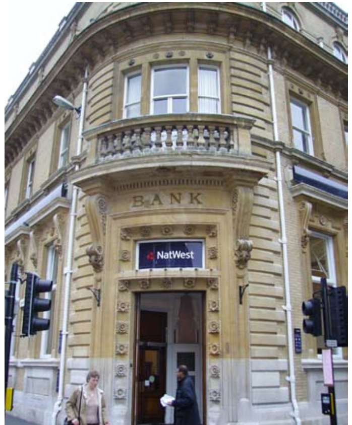
The impressive public entrance to the NatWest bank premises at the corner of Granby Street and Horsefair Street.
