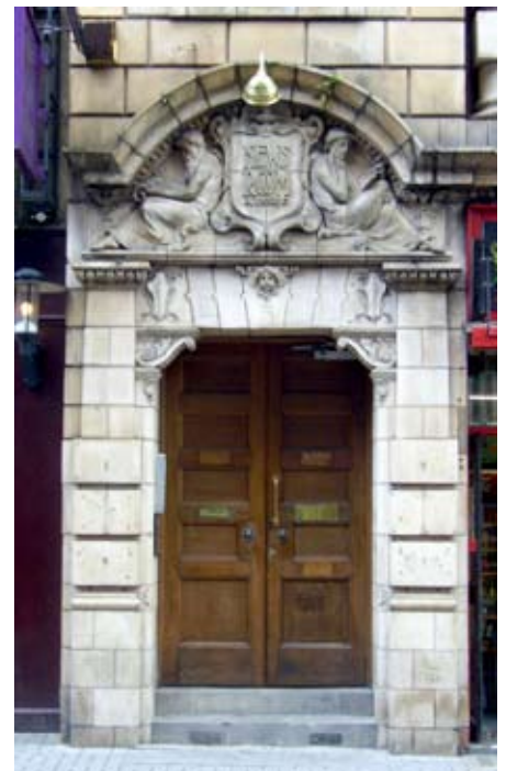
Detail of entrance to former General Newsroom, Belvoir Street.
