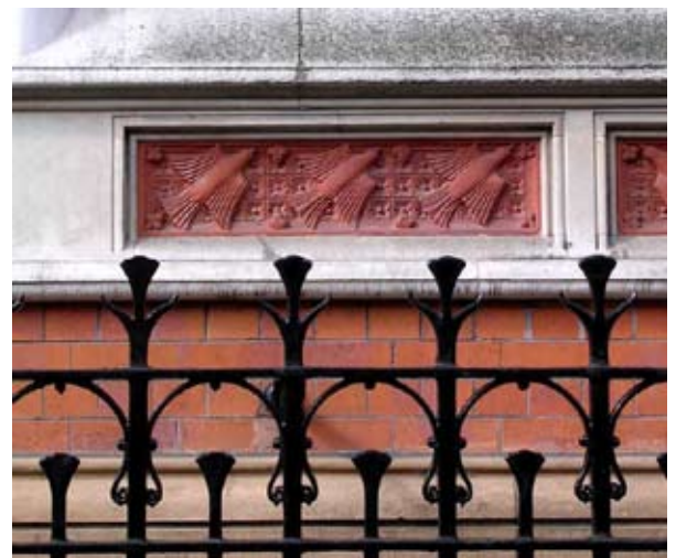
A detail of the moulded terracotta bird shapes and decorative ironwork to 31 Granby Street.
