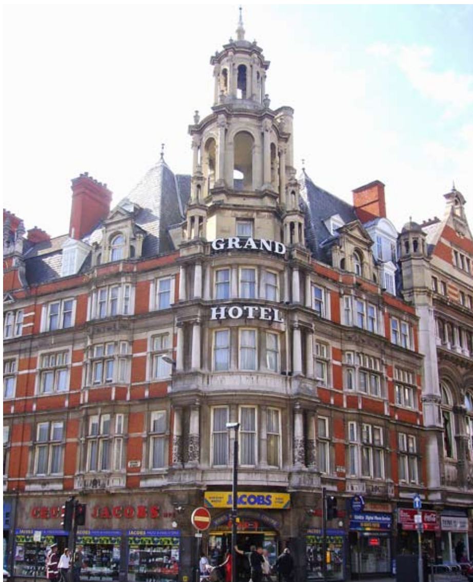
Granby Street/Belvoir Street corner is dominated by the tower of the Ramada Jarvis Grand Hotel. The architects may have been inspired by the churches of Sir Christopher Wren.
