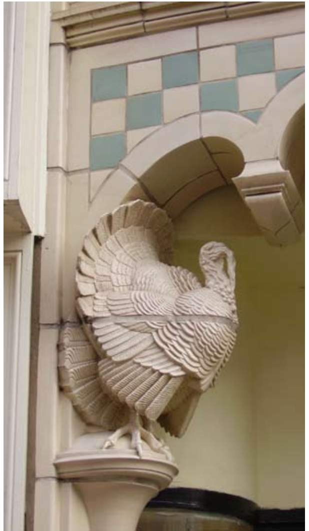
One of the two replacement "Turkeys" produced by Hathernware Ceramics of Loughborough for the 1984 restoration of the Turkey Café.
