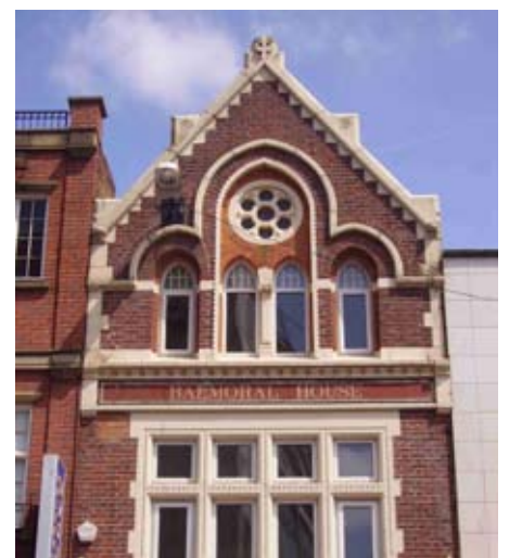
A close-up of 'Balmoral House', 88 Granby Street; it dates from 1873 and was designed by local architects Shenton and Baker
