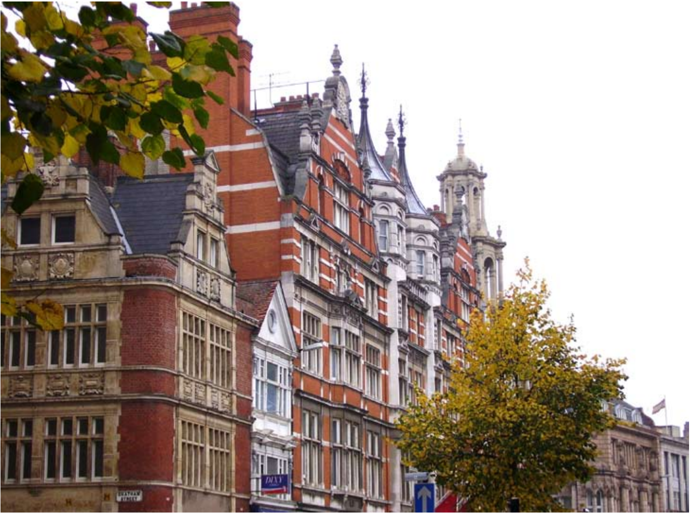
The range of architectural styles along Granby Street is exceptional. Here at the corner of Chatham Street the chosen style was Flemish, adjoining is the Grand Hotel with its varied skyline.
