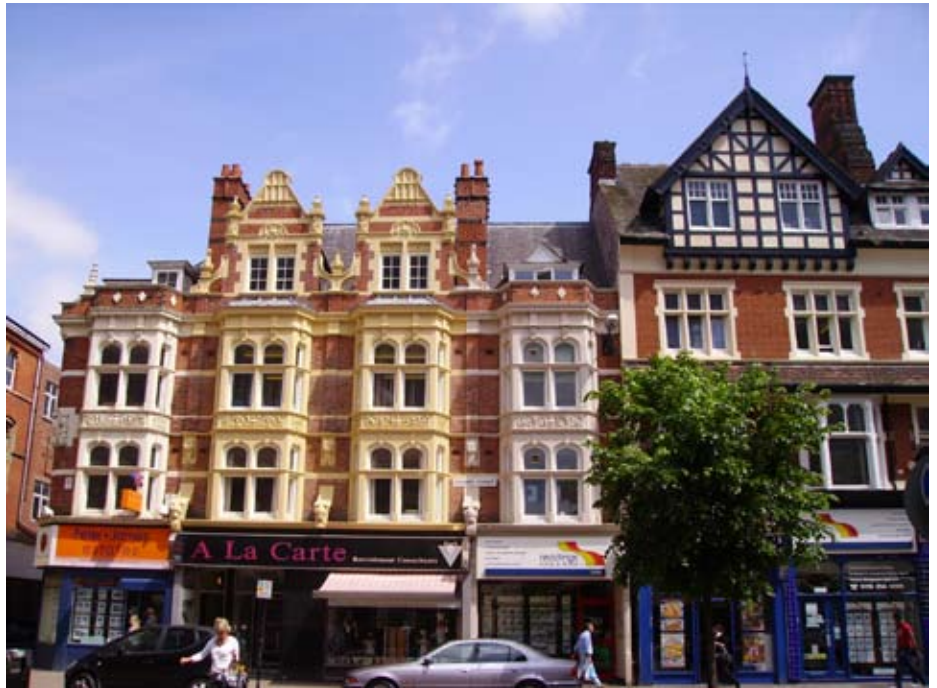
Numbers 76-82 Granby Street at the corner of Alfred Place combines a range of architectural styles and features a series of decorative carved brackets supporting the stone fascia.
