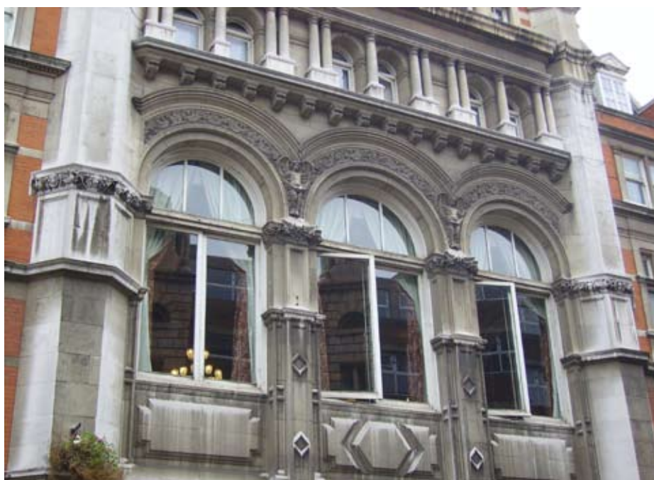
Part of the Belvoir Street elevation of the Ramada Jarvis Grand Hotel showing the three round-arched windows to the first floor ballroom/function room.
