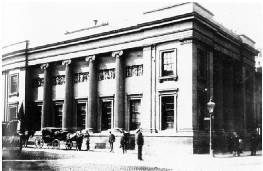
A view of William Flint's General News Room of 1838, this was certainly Flint's finest building but was unfortunately lost when Granby Street was widened in 1897/8.
