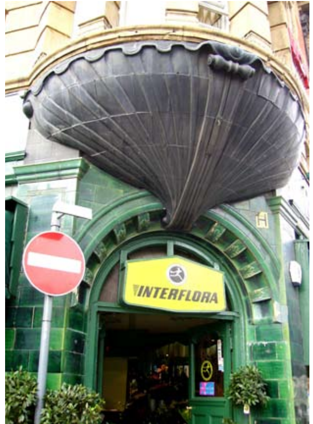
179 Granby Street, (part of YMCA). East Street corner of building showing entrance detail in green glazed tiles.
