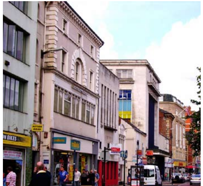
Only the upper, top two floors of Thomas Cook's Temperance Hotel at 123 Granby Street remain intact. Both the shopfront and first floors having been altered drastically. Beyond can be seen the large Portland stone building that was originally the Maples furniture store, built in the 1950s.
